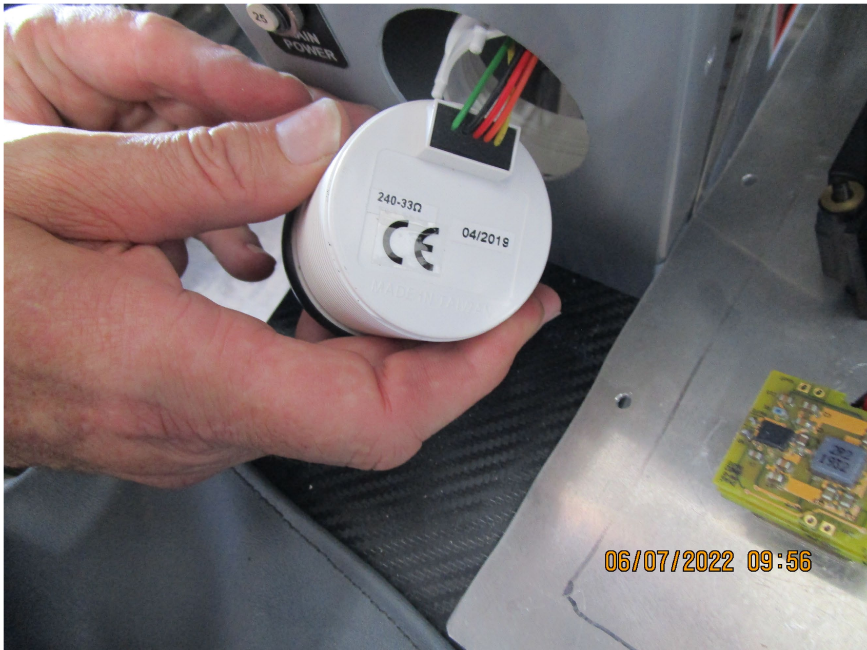
Photo 4 - Faulty fuel gauge (photograph provided by FAA)
