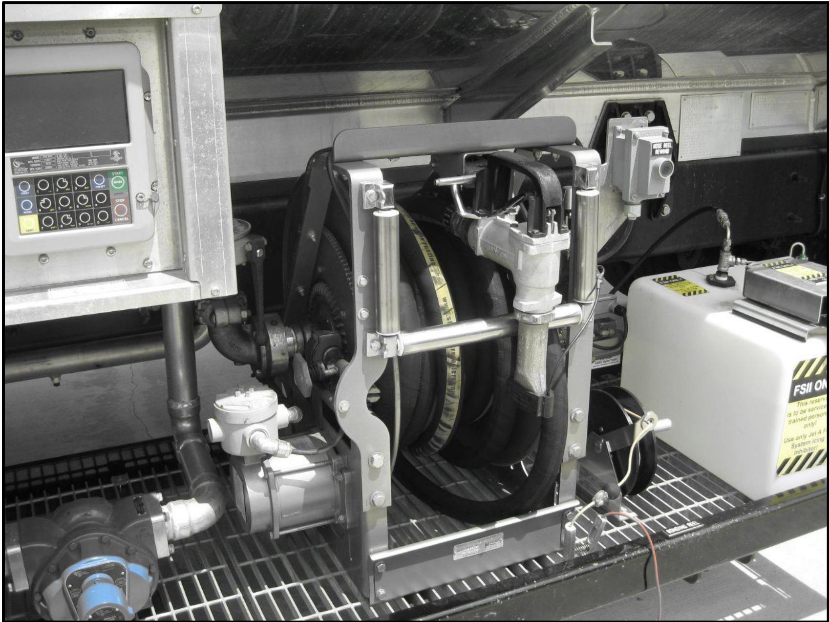
Photo 7 – Fuel Truck Hose/Nozzle (FAA Photo)
