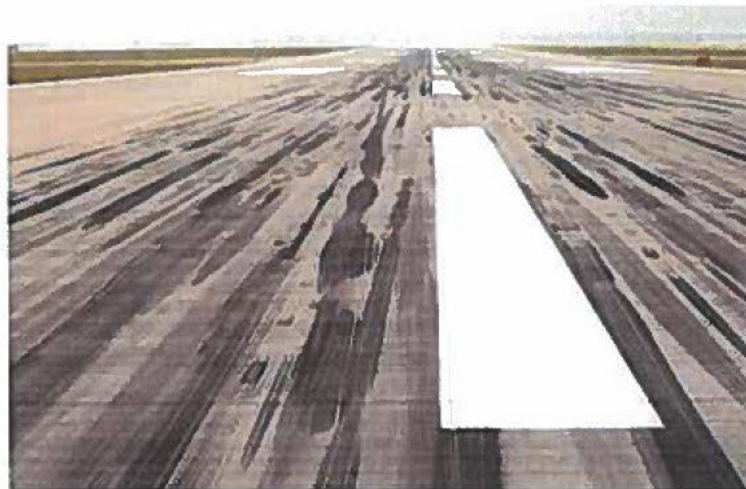
Figure 7: Example of tire marks showing rapid vertical oscillation of a tire (just left of runway centerline). (NOT the accident scene.)
