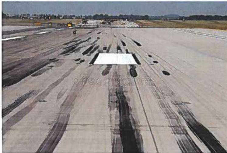
Figure 6: Examples of tire marks showing rapid lateral change of the tire direction (close to bottom of photo). (NOT the accident scene.)
