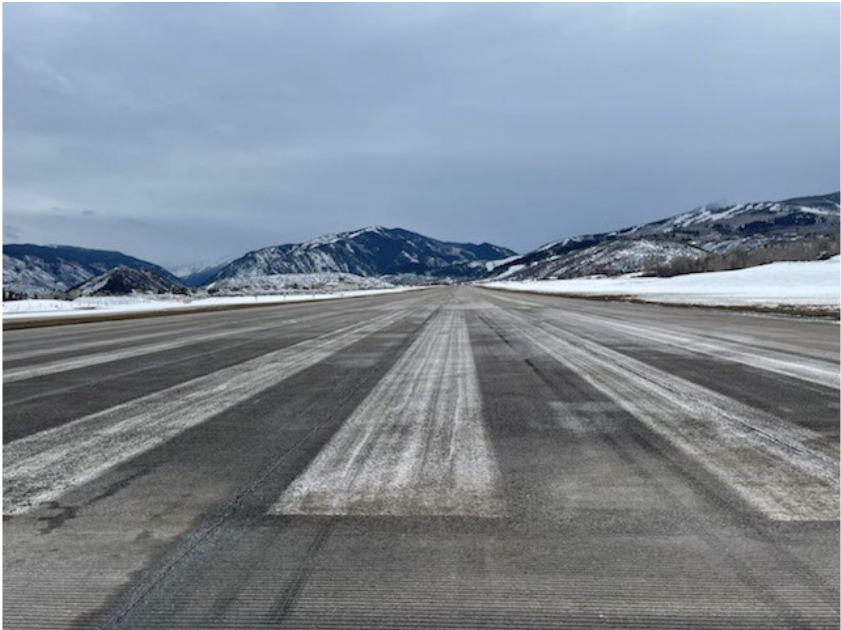
Photo 2 – Runway threshold South (Source: ASE Airport Operations)
