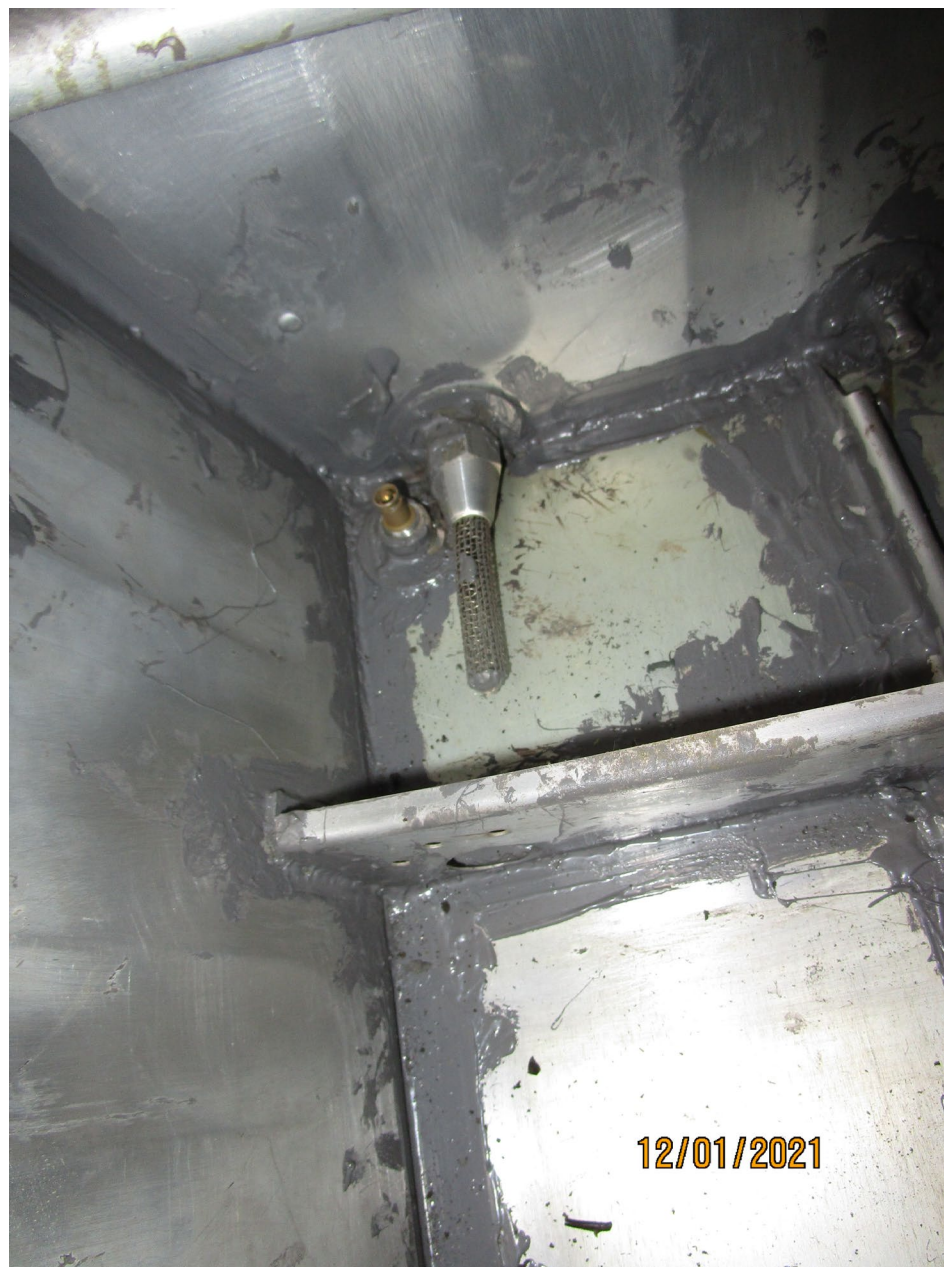
Photo 7 – View of the interior of the right fuel tank.
