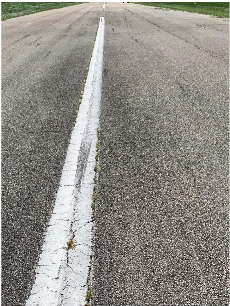
Photo 12 – First Impact Tire Mark
