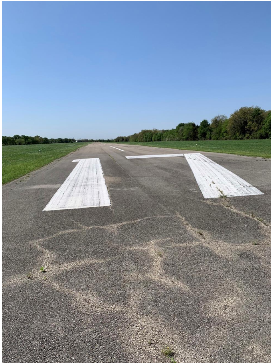
Photo 11 – Approach End of Runway 17
