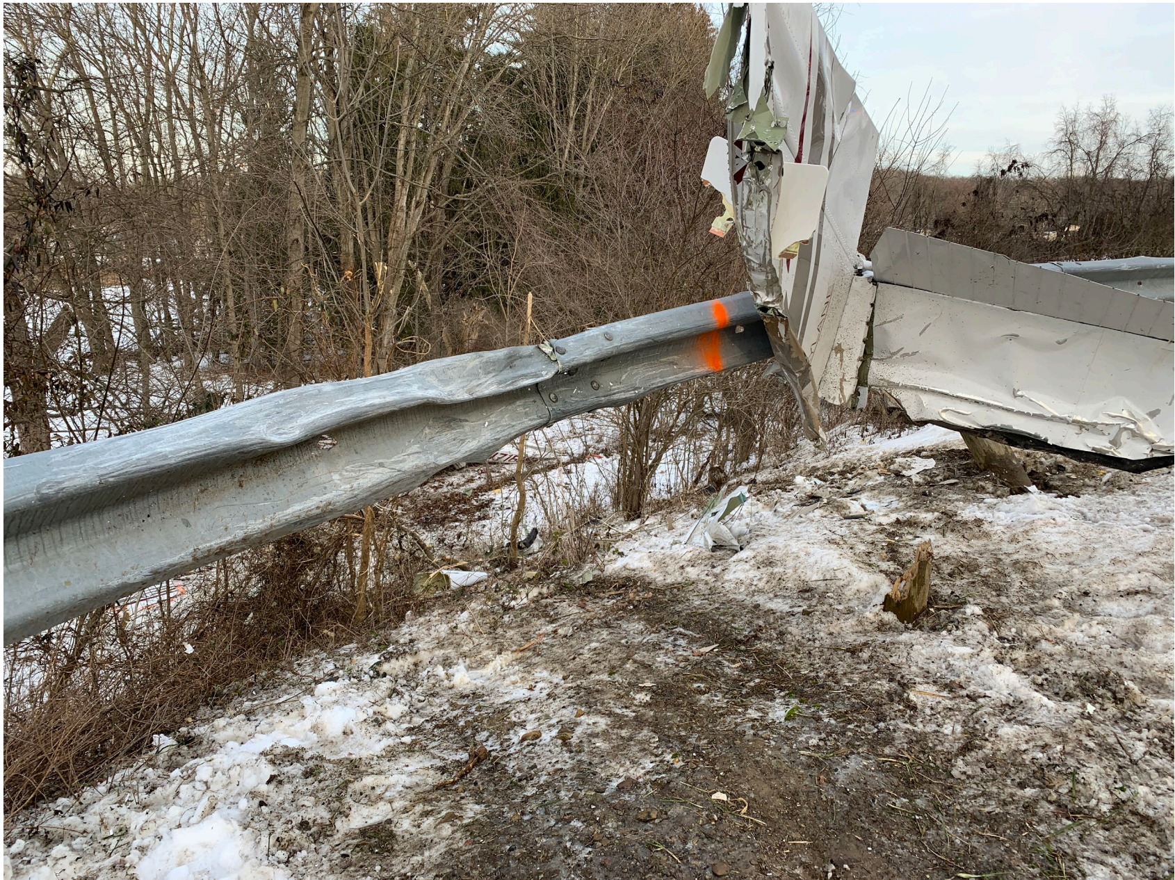
Photo 10 – Empennage Section (Source: NTSB)
