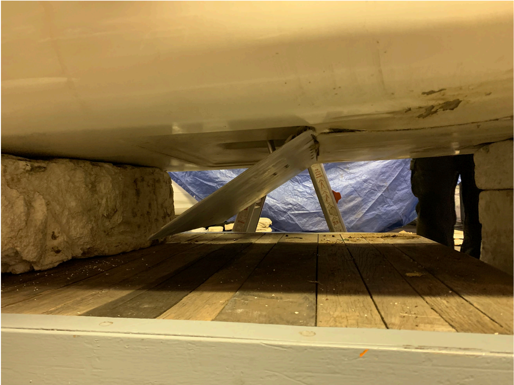
Photo 8 – View of the extended air brake, showing the bottom of the panel.
