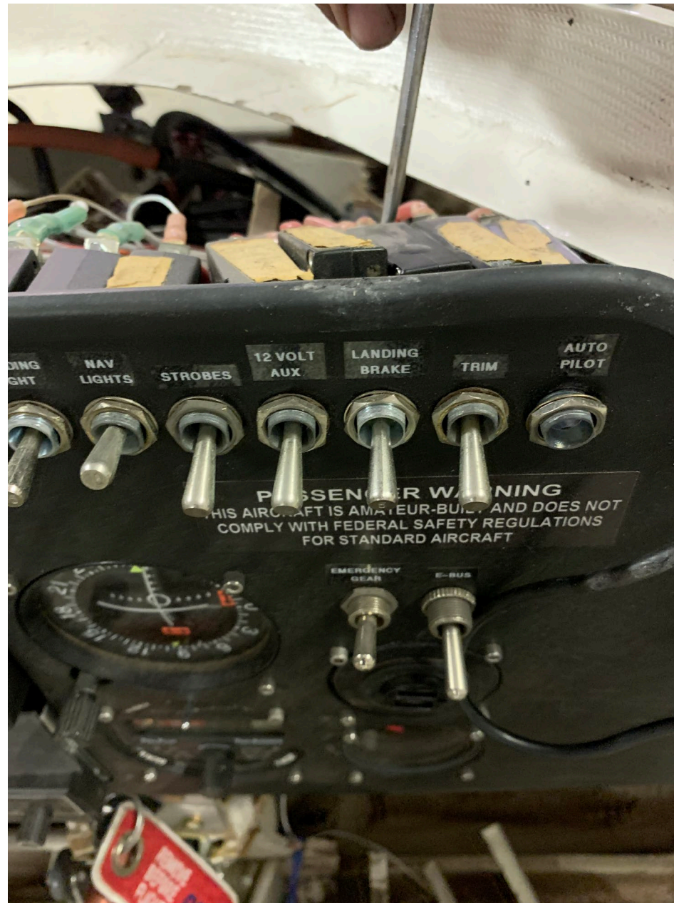
Photo 12 – View of the landing brake switch.
