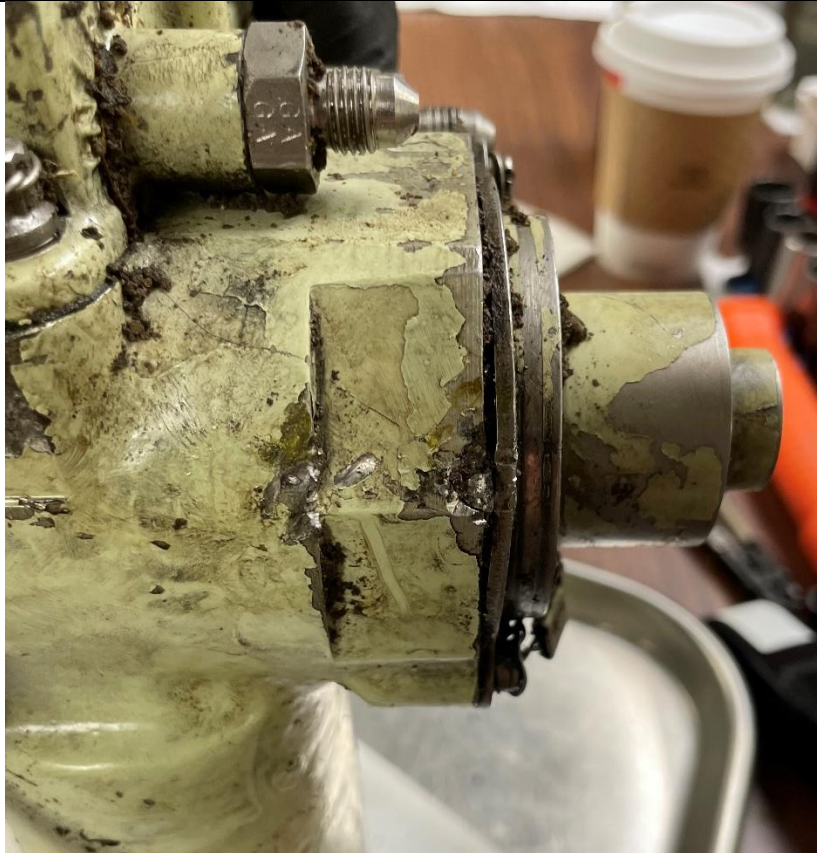
Figure 1. Damage to Housing
