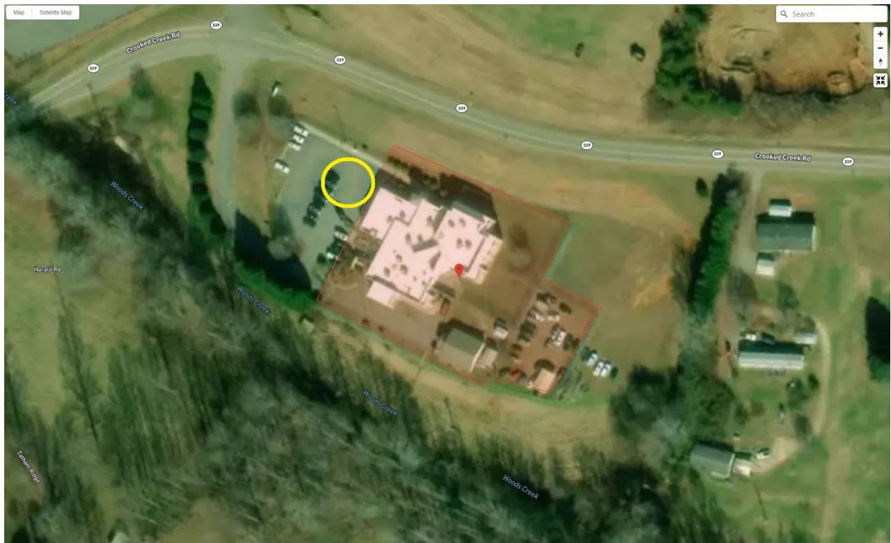
Figure 2. Restricted Zone highlighted in red and approximate accident location circled in yellow.
