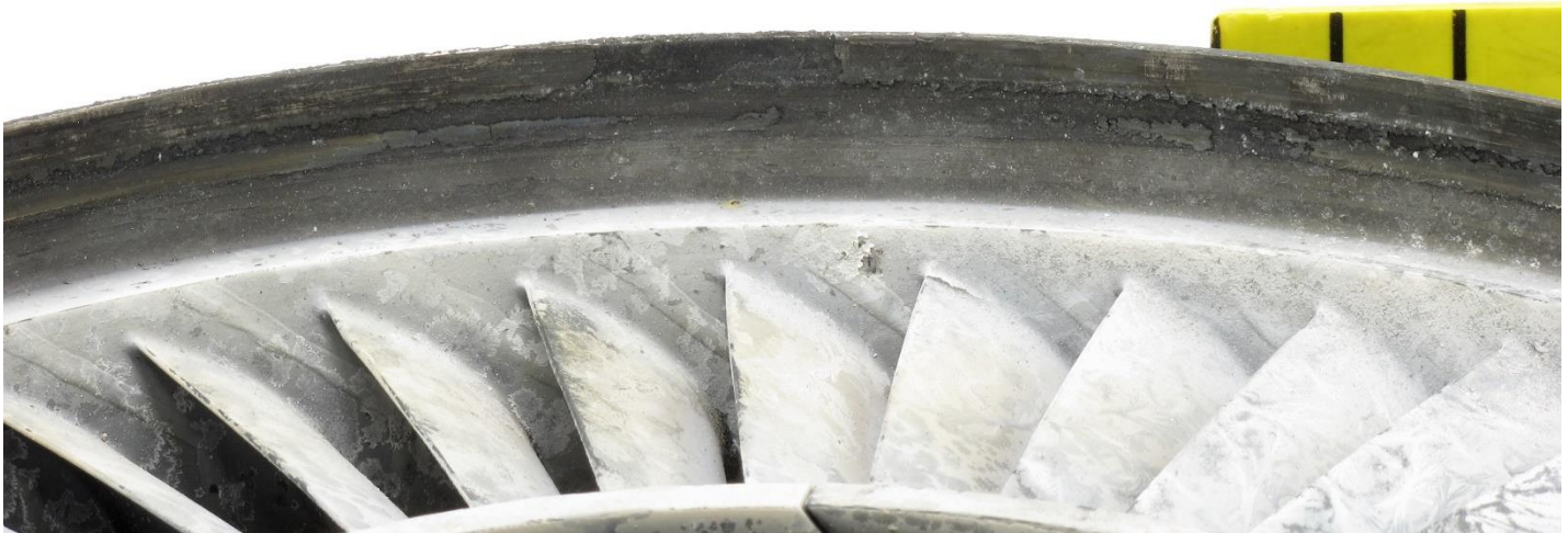
Figure 71. Detailed views showing the fourth stage turbine blade track in the fourth stage turbine nozzle. The nozzle was rotated 90° counterclockwise (FLA) for this succession of images. The blade track exhibited rub damage around the entire circumference. Divisions = cm.
