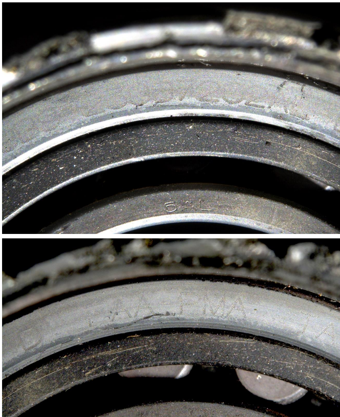
Figure 98. Detailed views showing the part number (top) and PMA (bottom) part markings on the No. 7 bearing. No scale provided.
