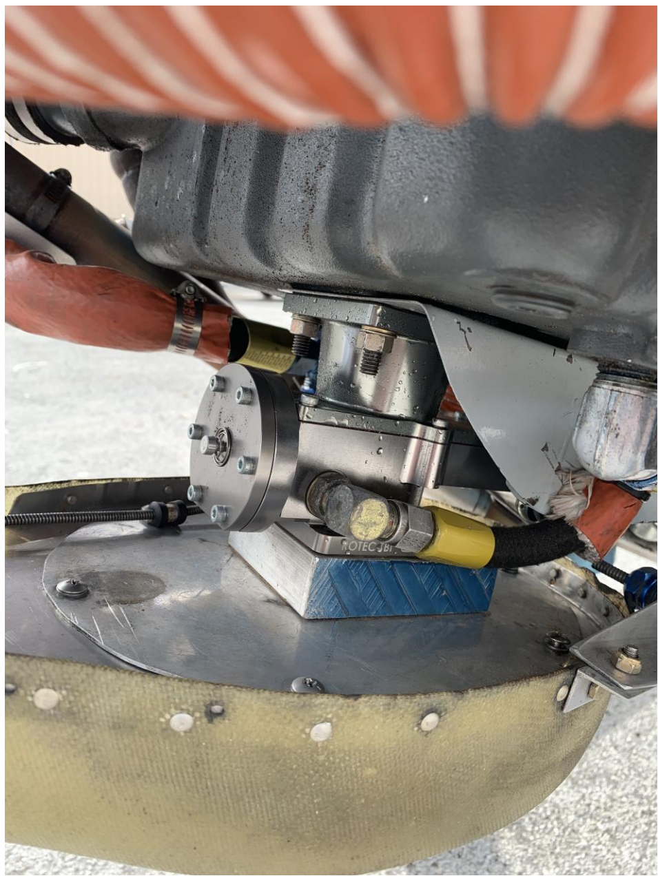
Photo 3 – Throttle Body Injector Installed
