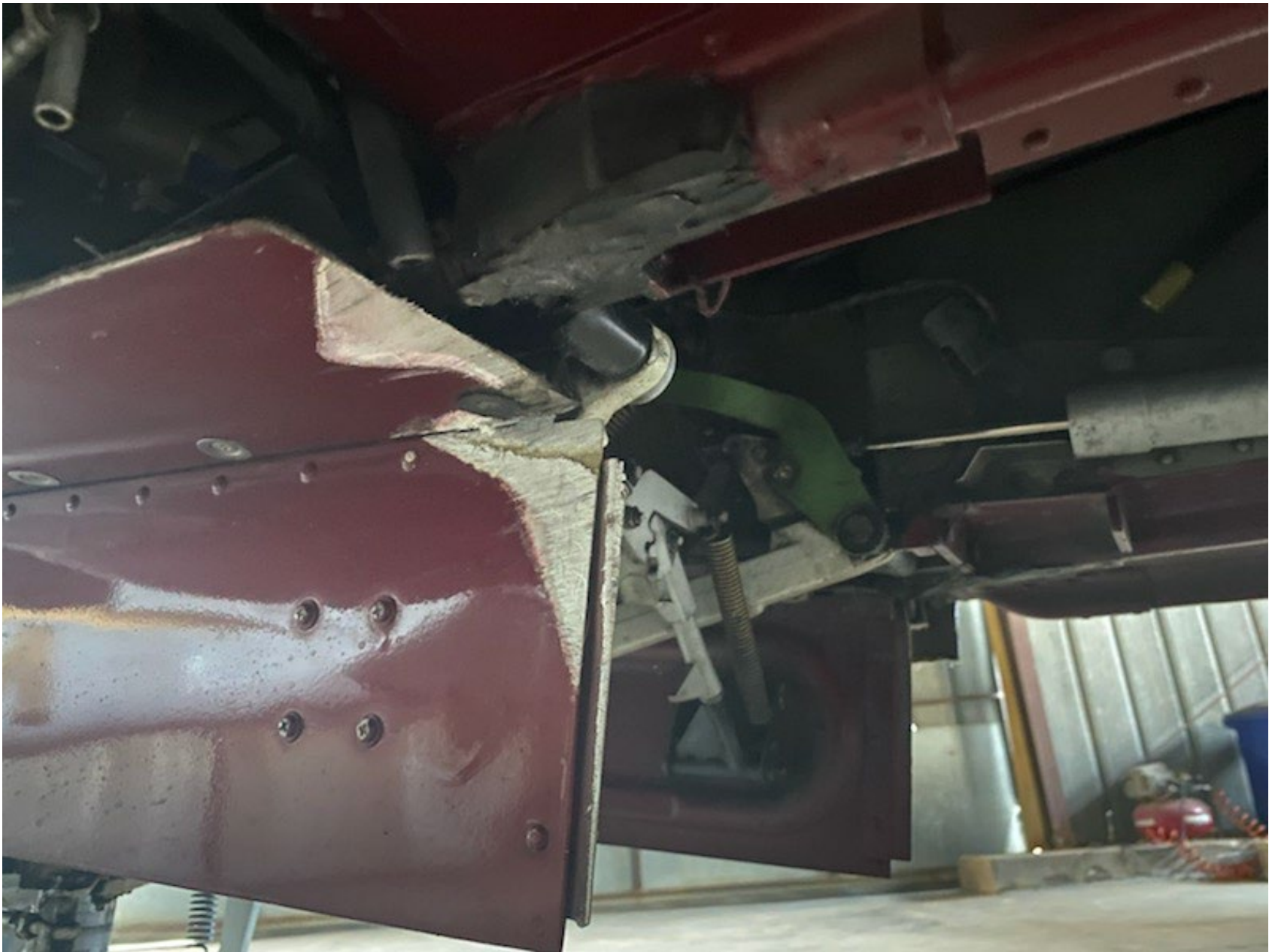
Photo 2 – Nose wheel landing gear bay (Provided by FAA)
