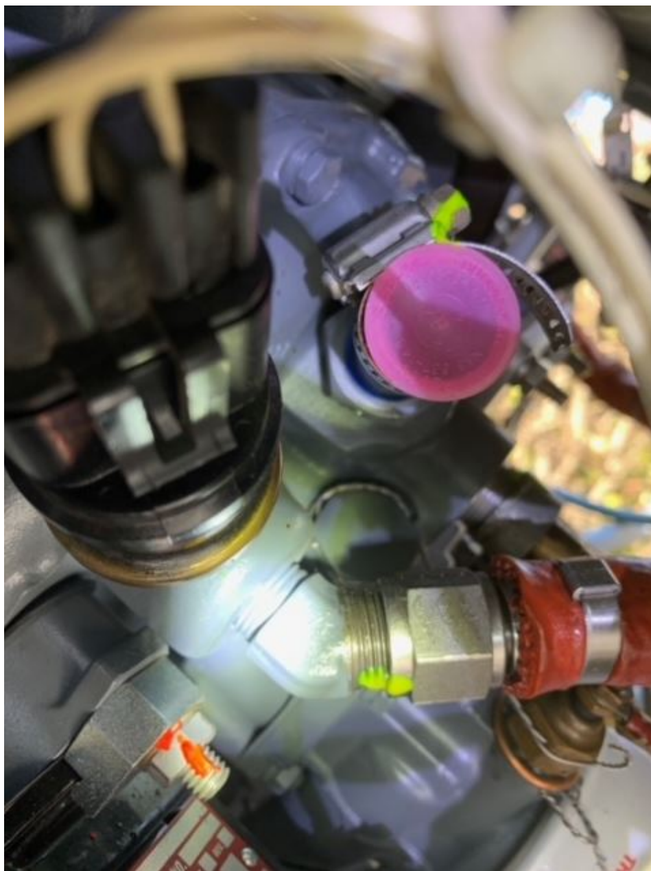
Photo 3 – Blocked Crankcase Breather Port (FAA Photo)
