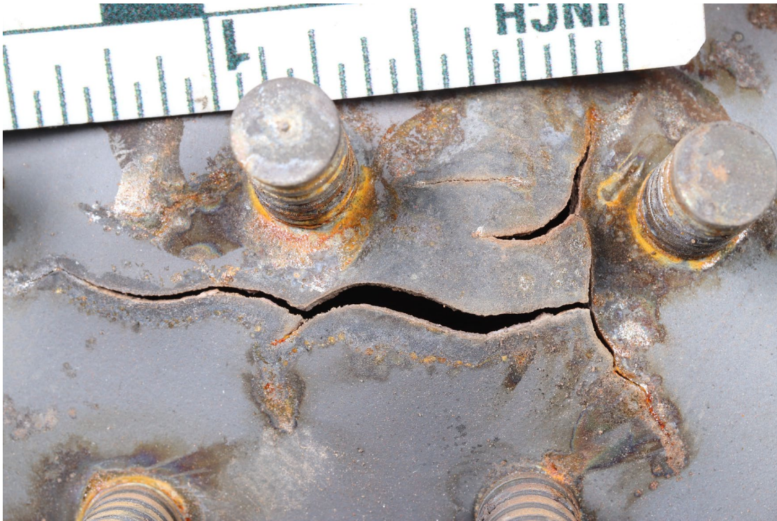
Figure 5: Branching cracks on the barrier between exhaust gas and cabin air.
