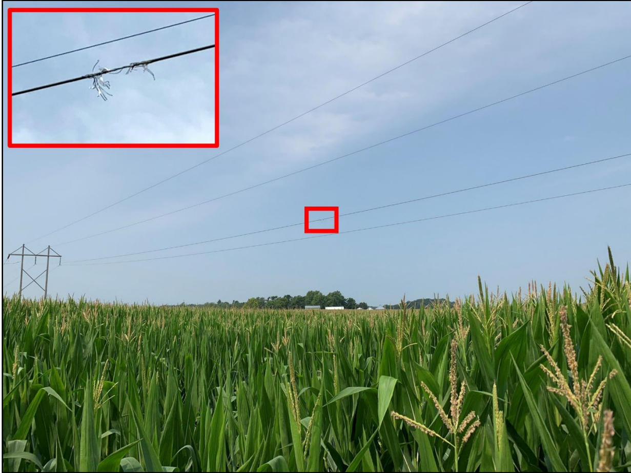
Figure 2. Power lines above the cornfield with a red rectangle identifying the center power line that was damaged during the accident. A separate closeup photo shows the frayed center power line in more detail.
