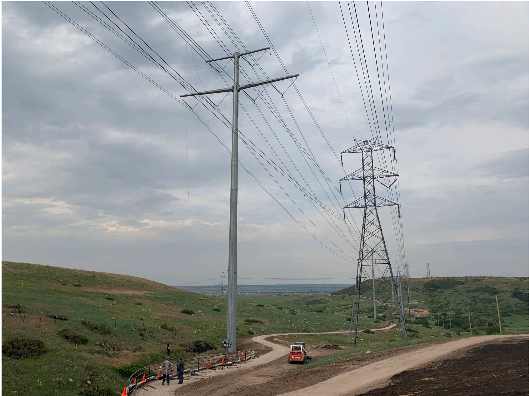
Photo 10 – View from underneath the transmission static lines.
