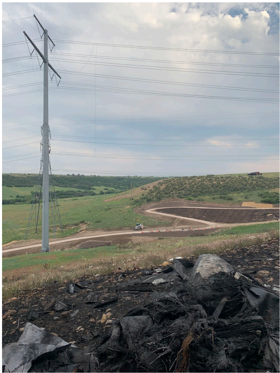
Photo 9 – View of the transmission static lines from the accident site.
