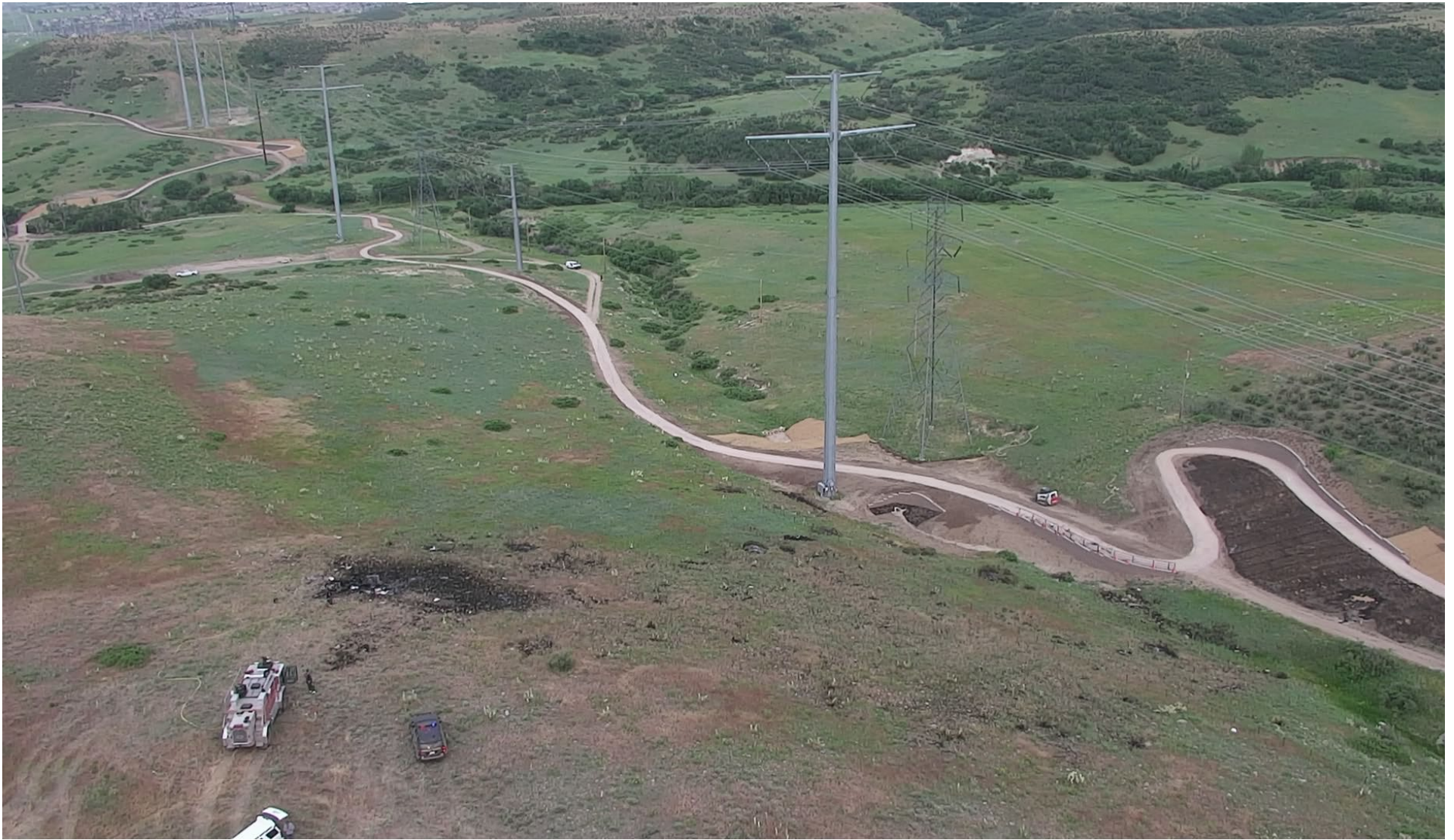
Photo 2 – Aerial view of the transmission static lines and the accident site, looking to the east (courtesy of the South Metro Fire Rescue Authority).
