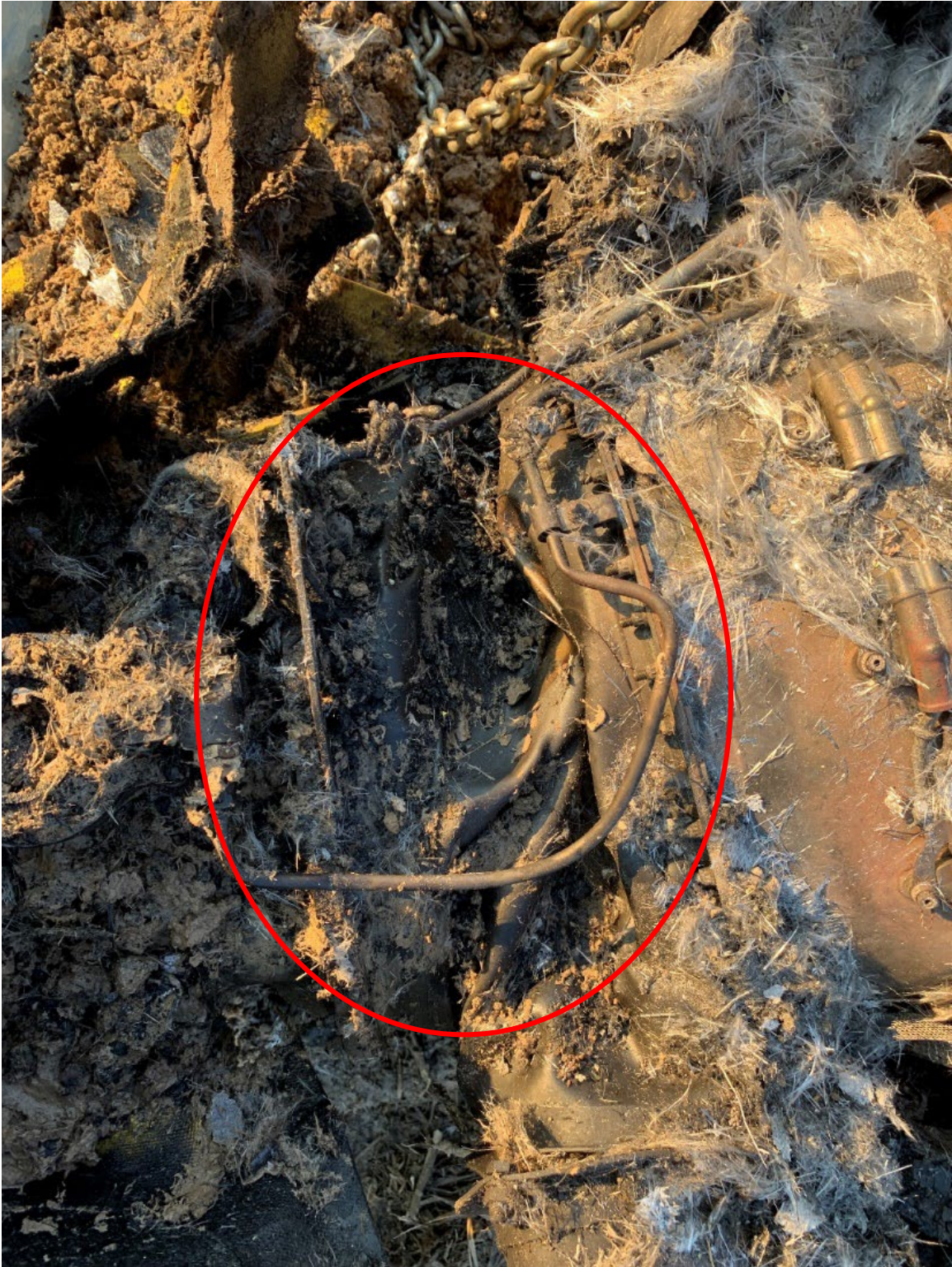
Figure 22: Deformation and Buckling on top of the Reduction Gear Housing.
