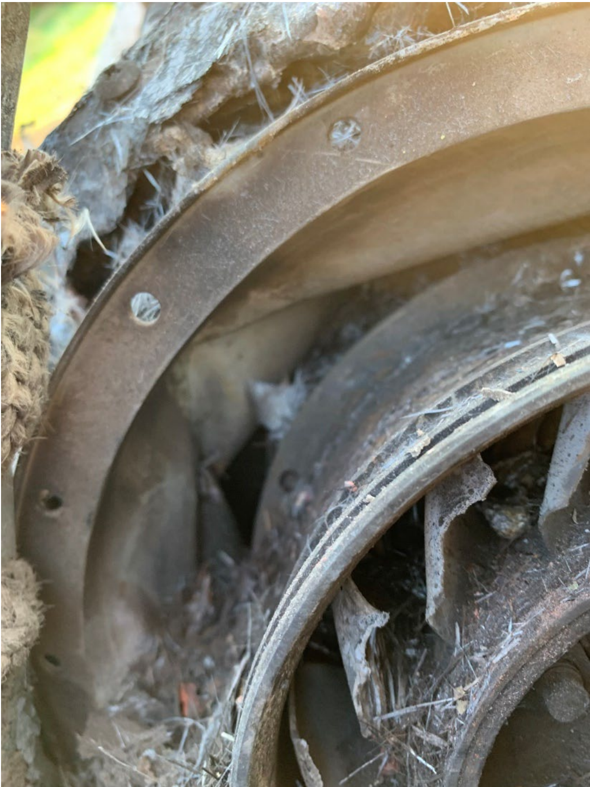
Figure 24: The First Stage Compressor
