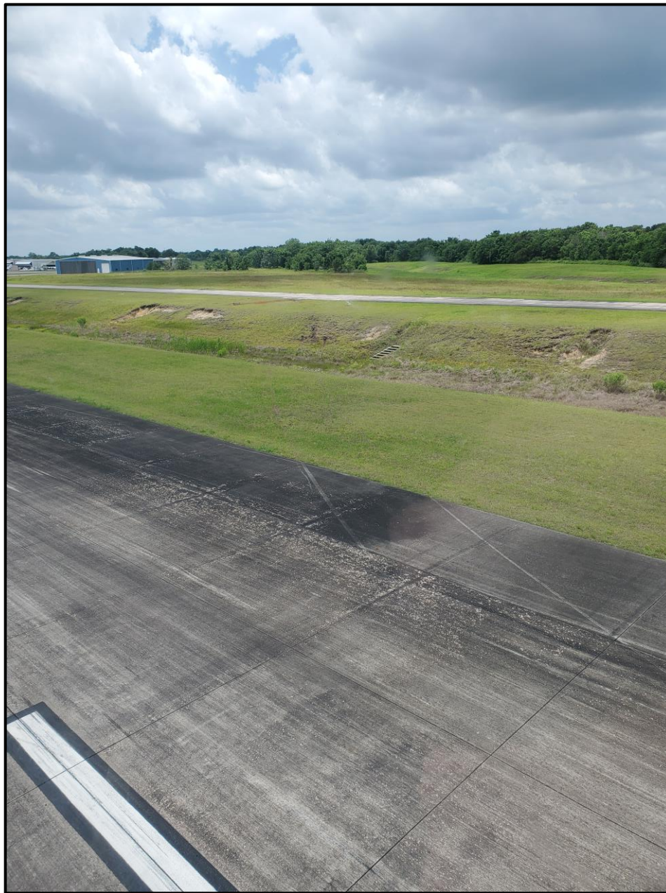
Photo 5 – Accident Site (Witness Photo)
