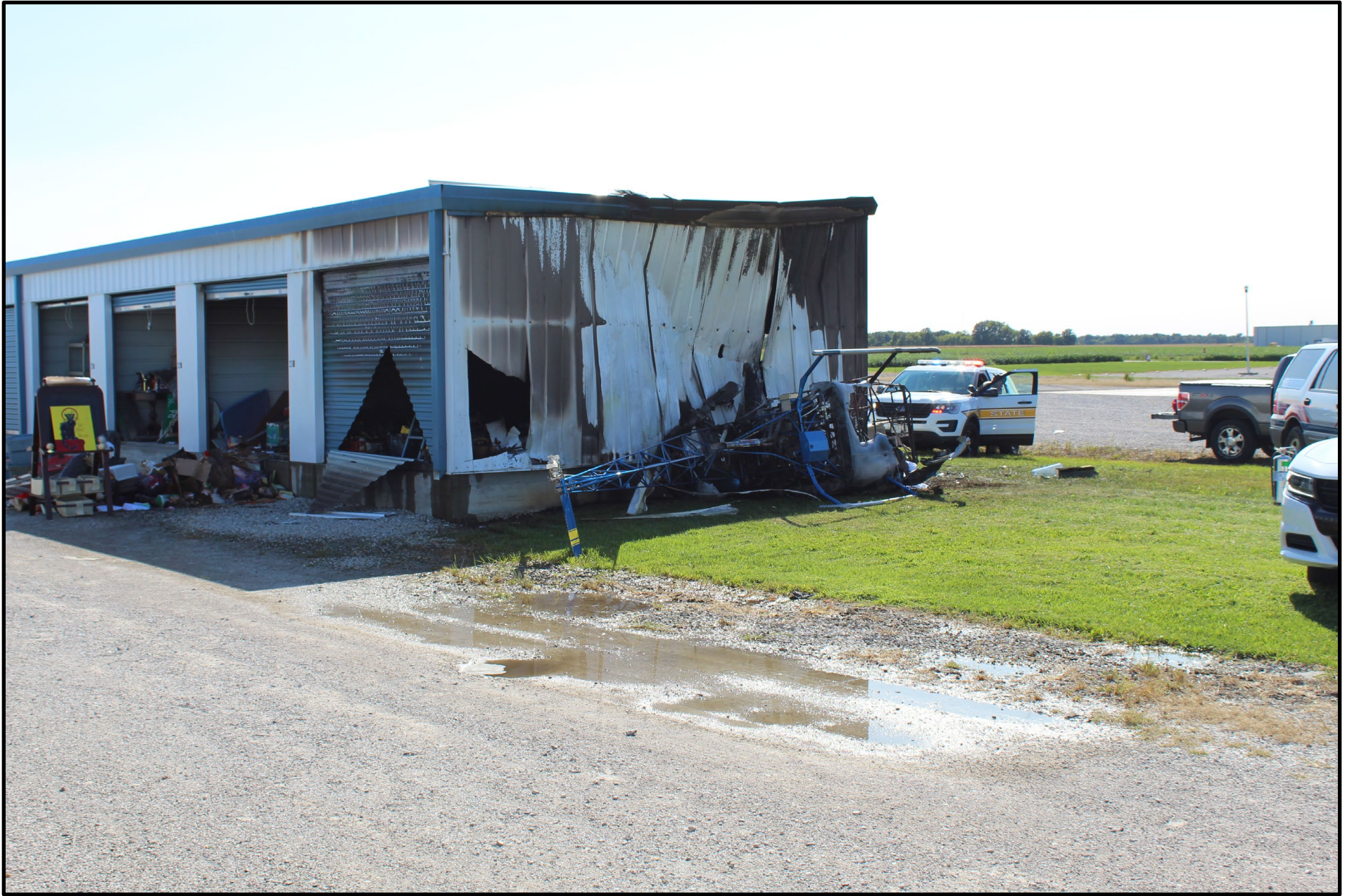
Photo 2 – Accident Site (State Police Photo)
