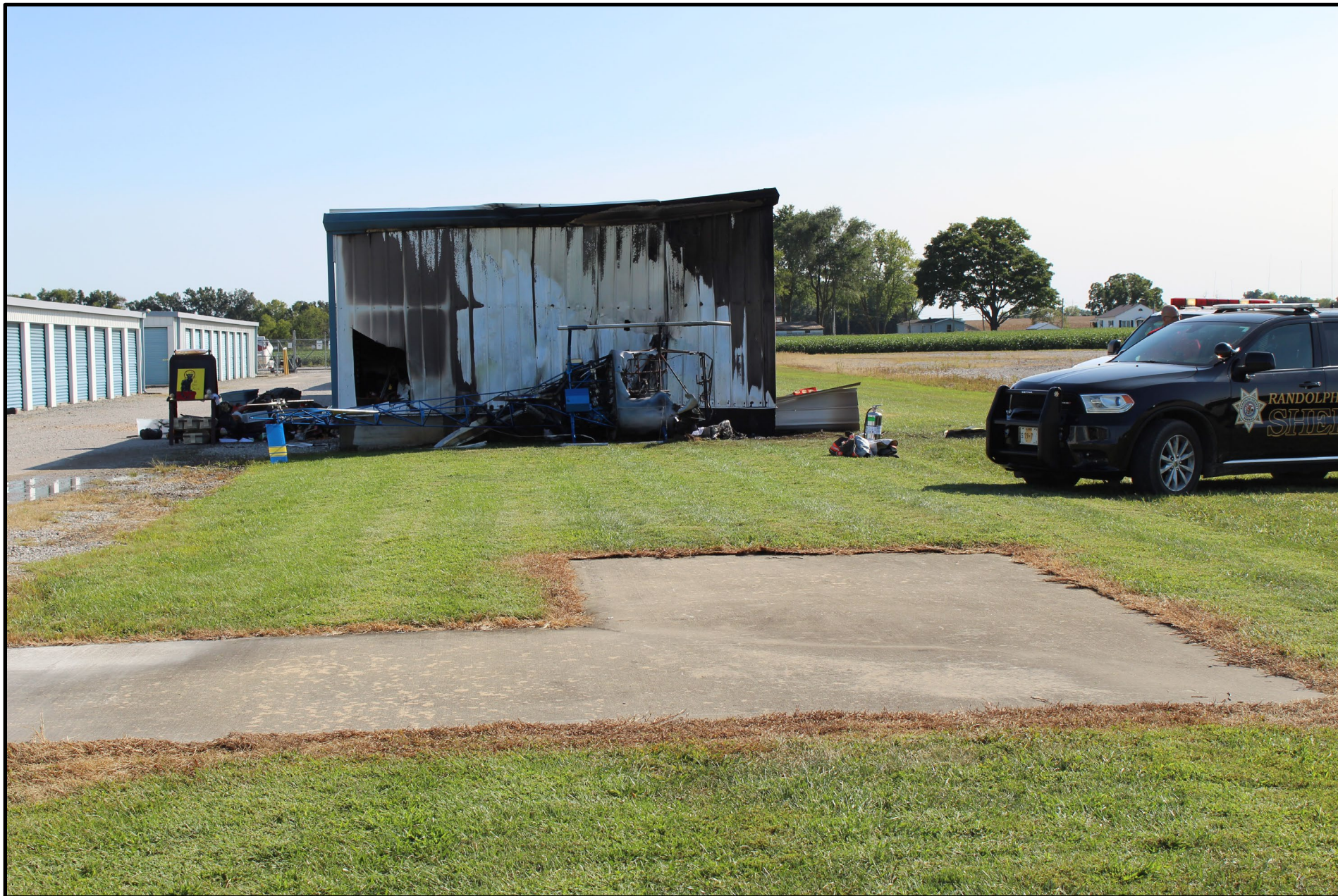
Photo 1 – Accident Site (State Police Photo)
