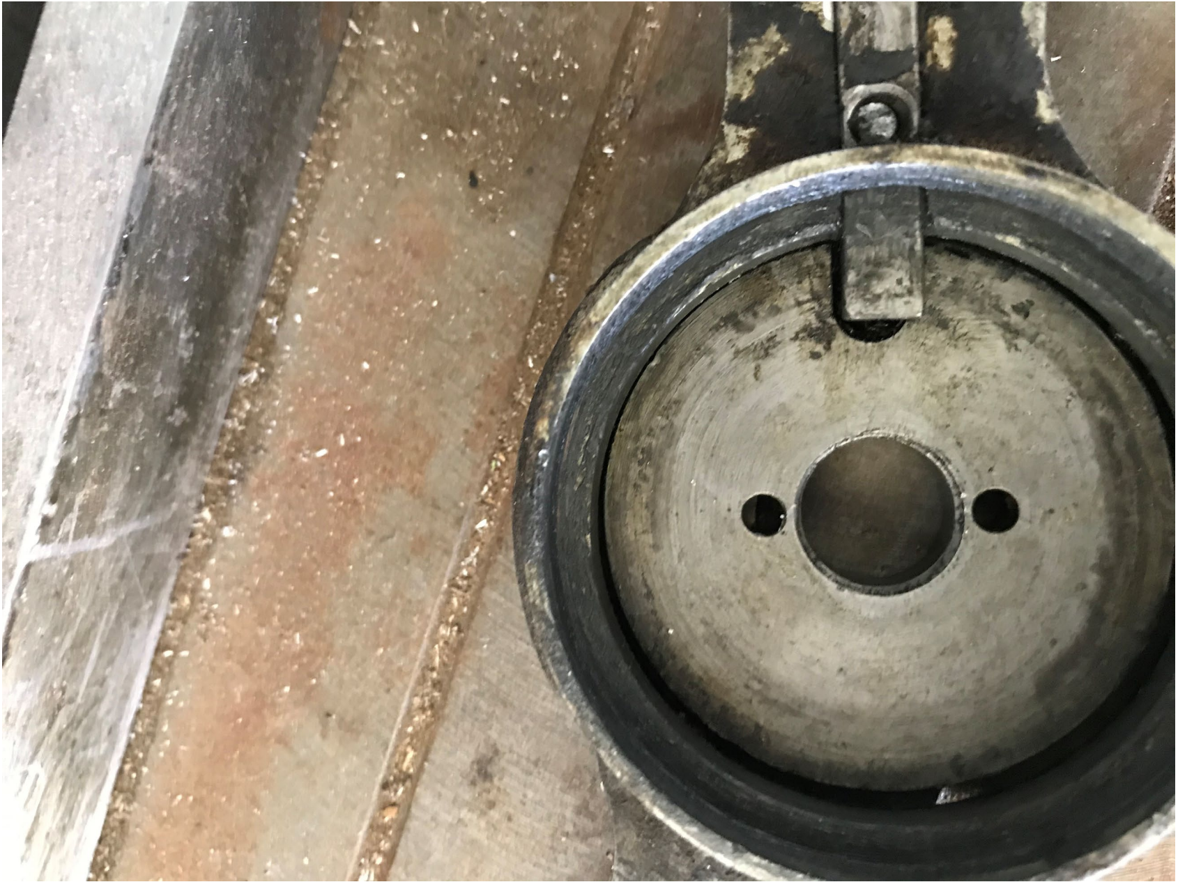
Photo 3 – Accident Locking Pin Assembly
