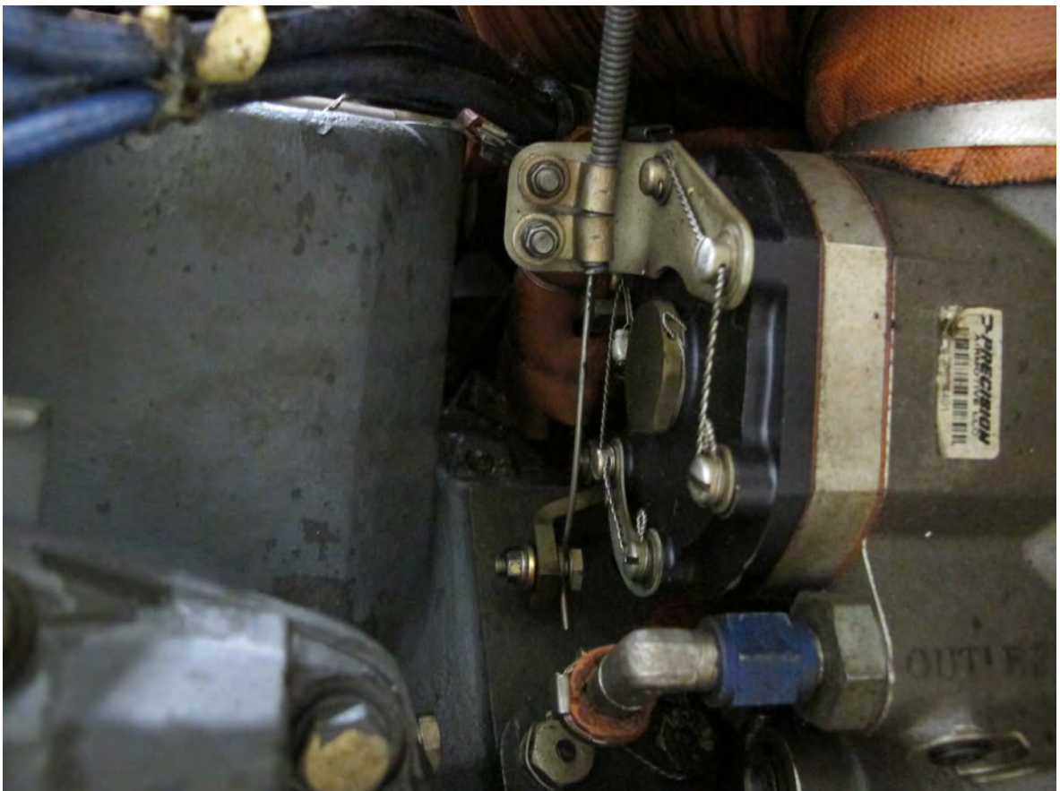
Fuel mixture control at fuel control unit.
