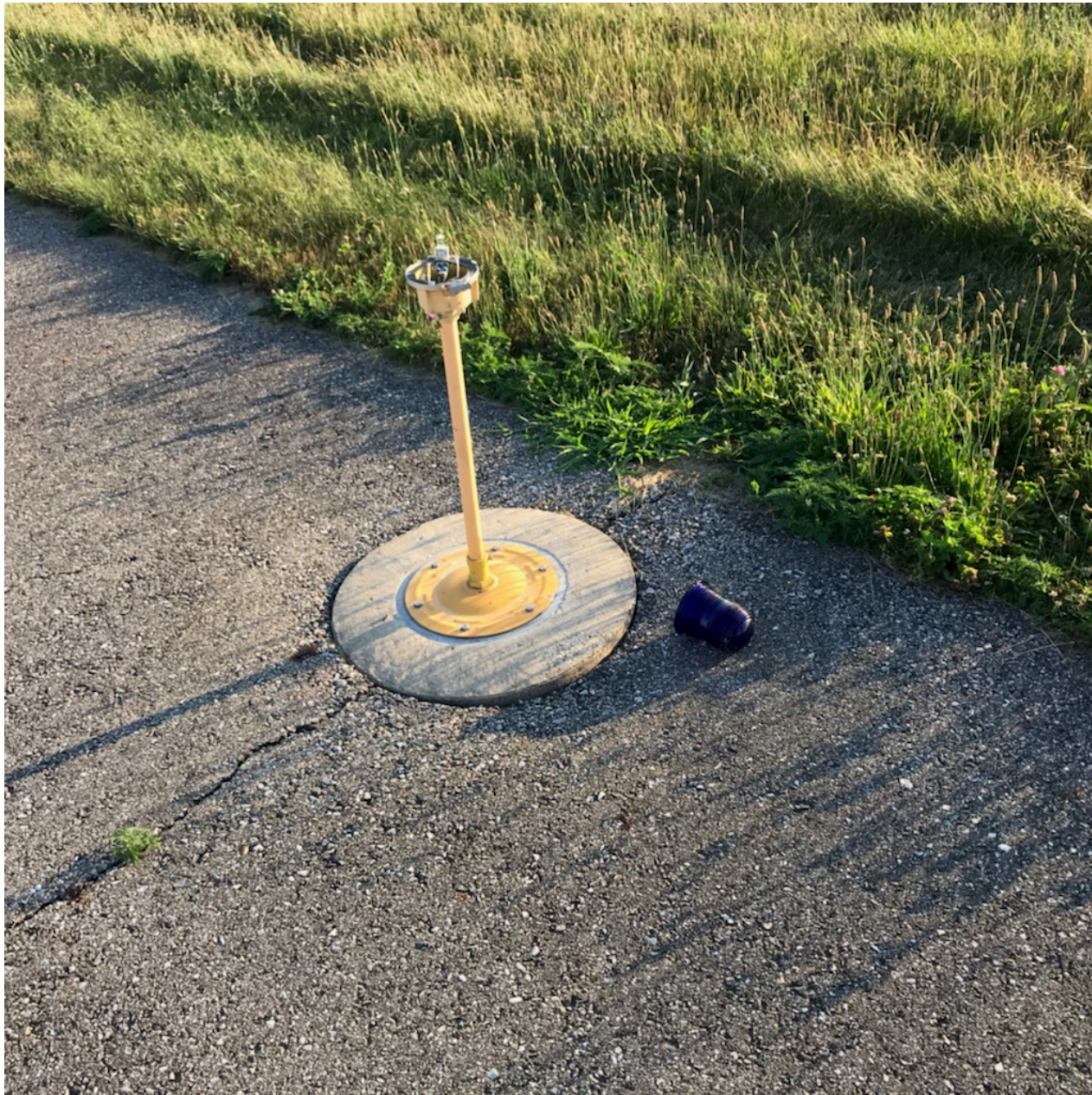
Photo 2 – Taxiway light struck by N50JH during takeoff, located at intersection of taxiways C and E (FAA photo)
