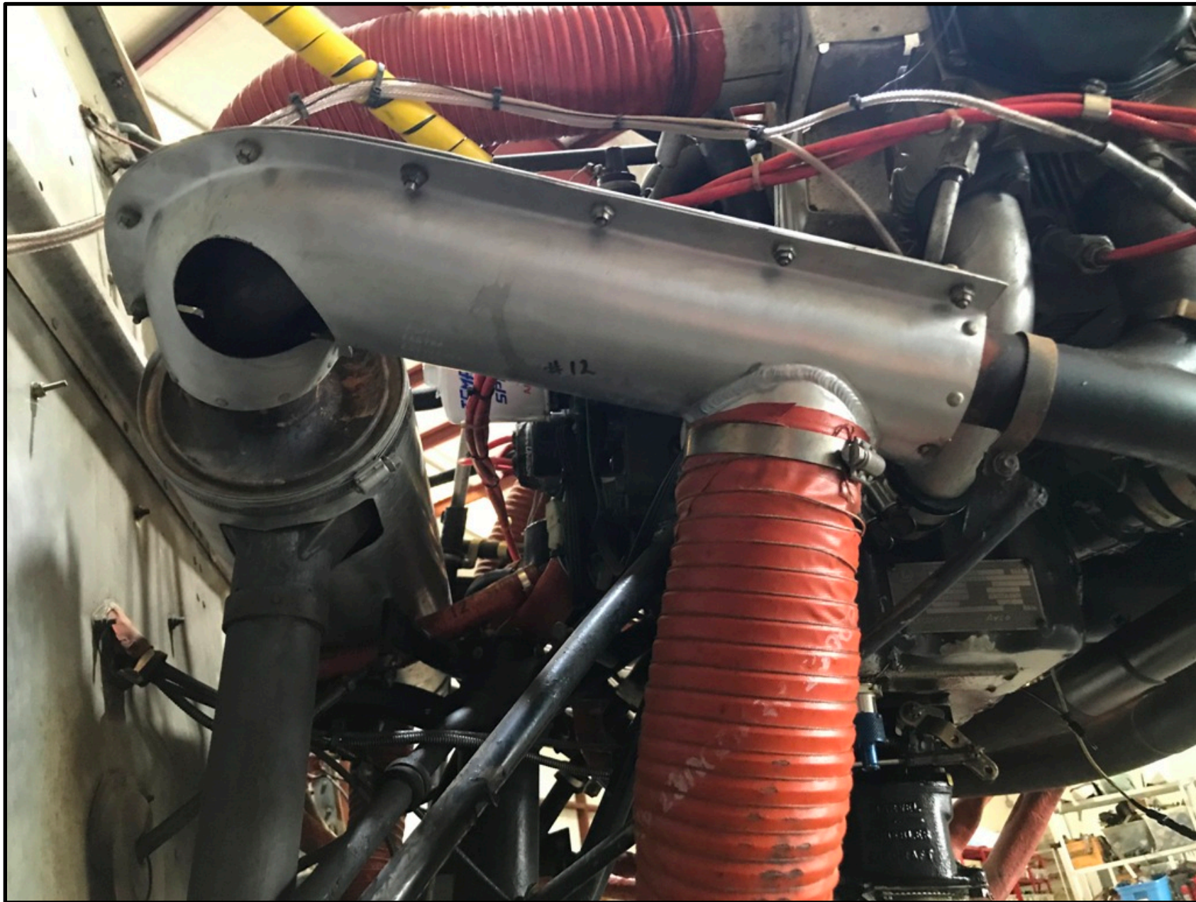
Photo 5 – Carburetor Heat Shroud -- Duct
