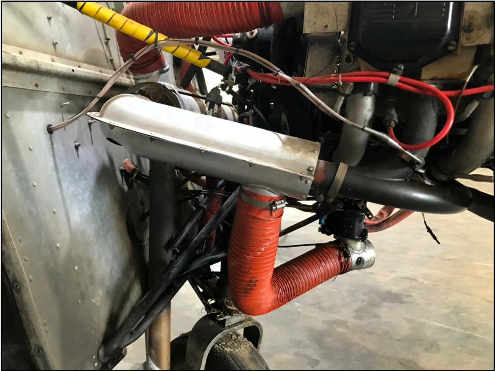
Photo 4 – Carburetor Heat Shroud -- Duct
