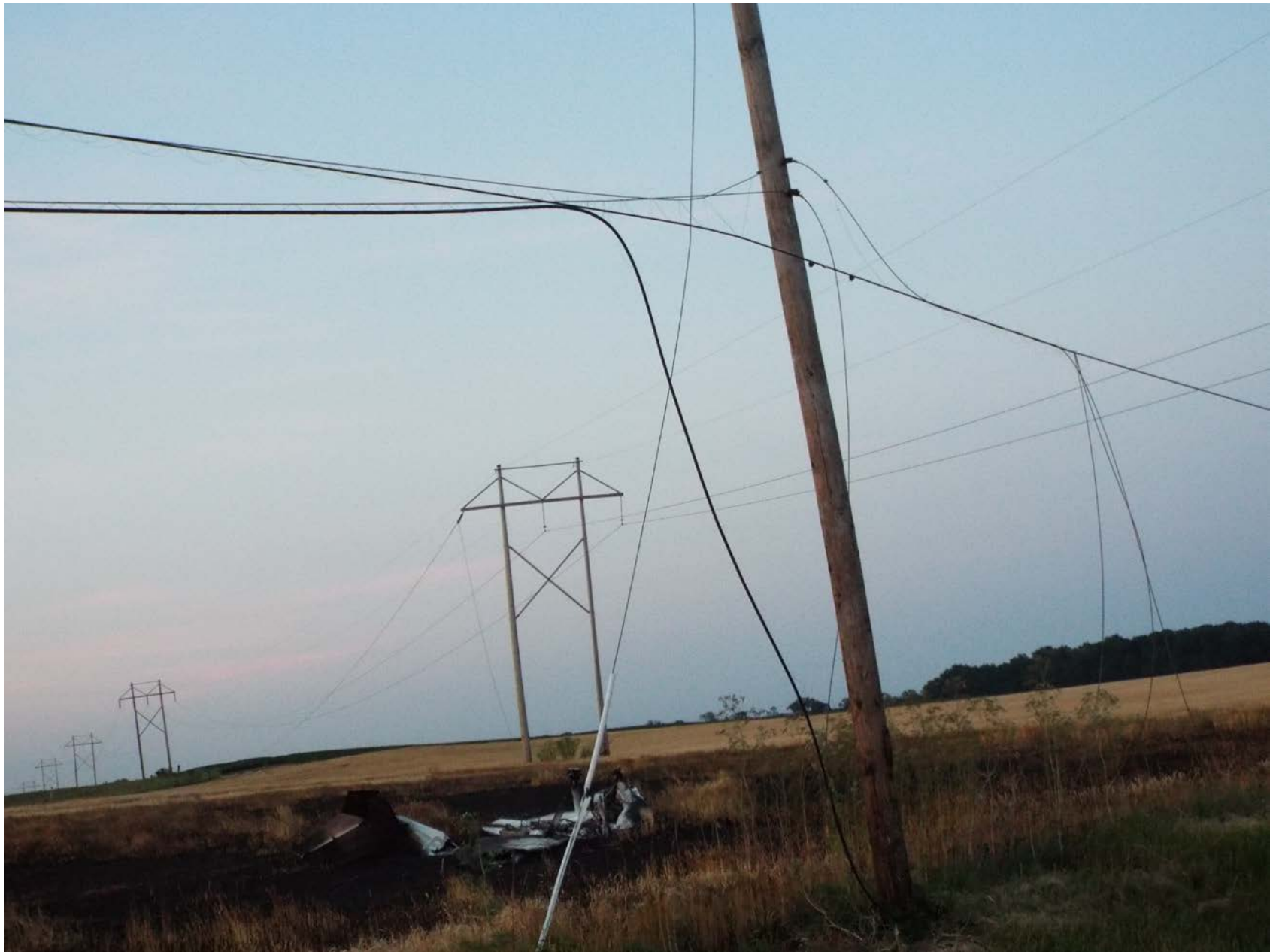
Photo 2 – Downed power lines, airplane wreckage in background (FAA photo)
