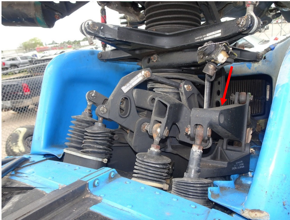
Figure 15. Transmission deck flight control bellcranks. The red arrow points to the directional control system bellcrank at STA 96.
