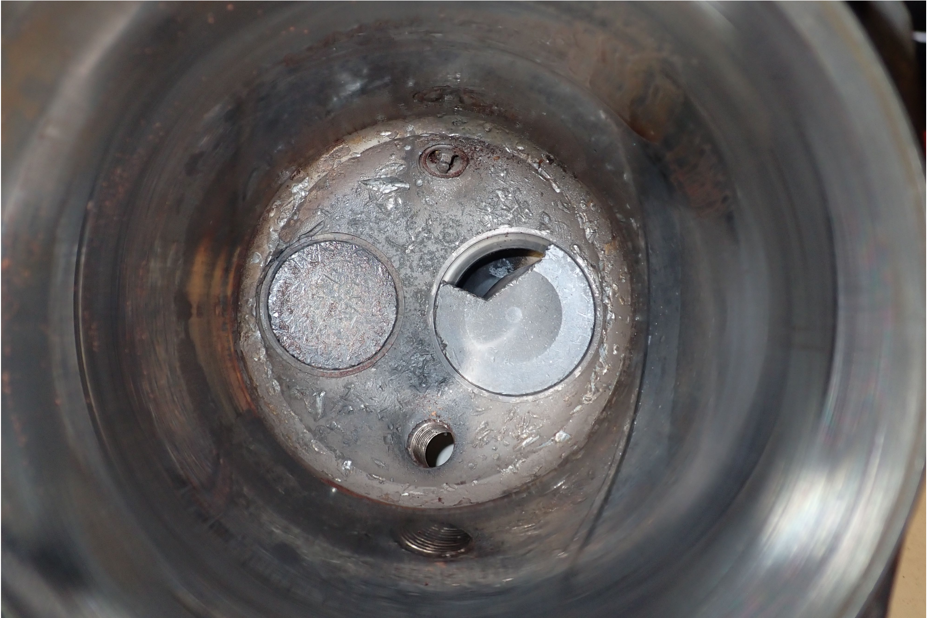
Photo 7 – Inside No. 1 Cylinder
