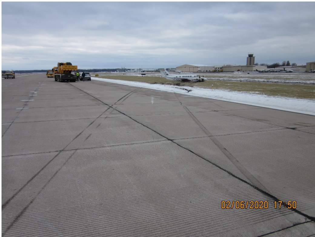
Figure 2: Skid Marks on Runway Leading Off Pavement to Right (Courtesy of FAA)
