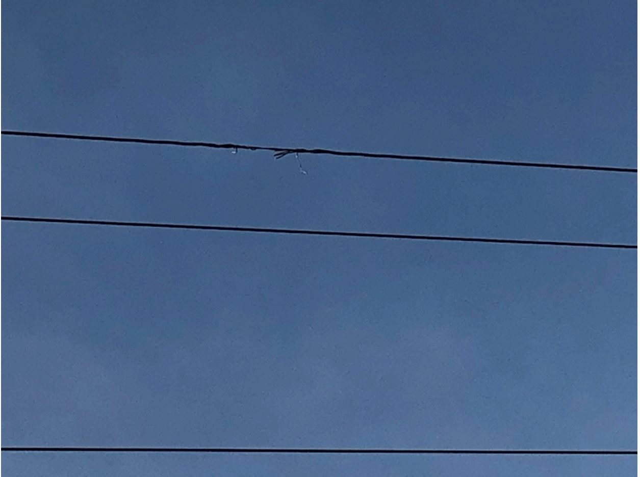
Photo 3: Damaged Powerline
