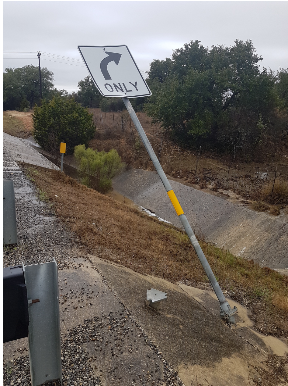
Photo 2 – Roadway Sign Stuck by Airplane
