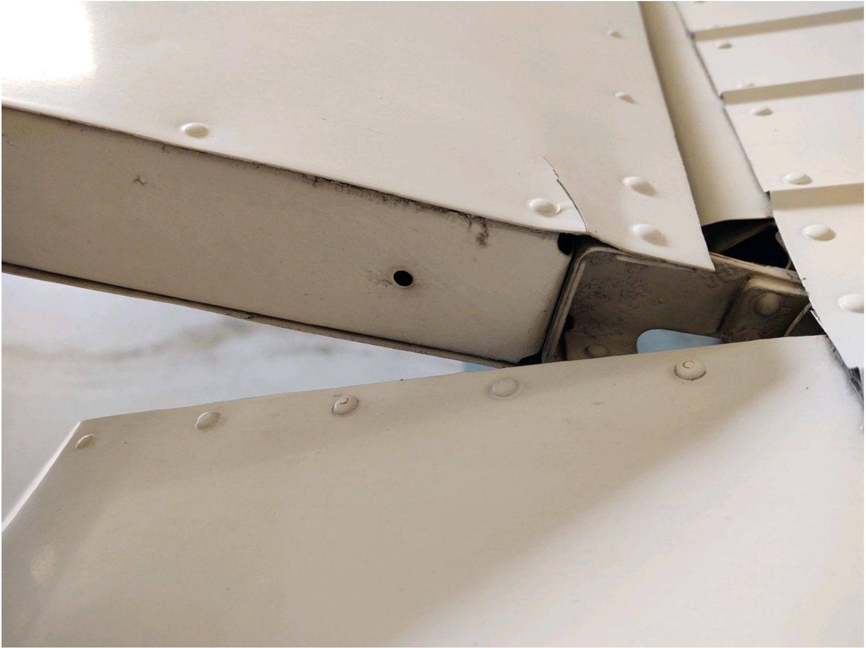
Photo 3 – Left Elevator (Purdue Aviation Photo)
