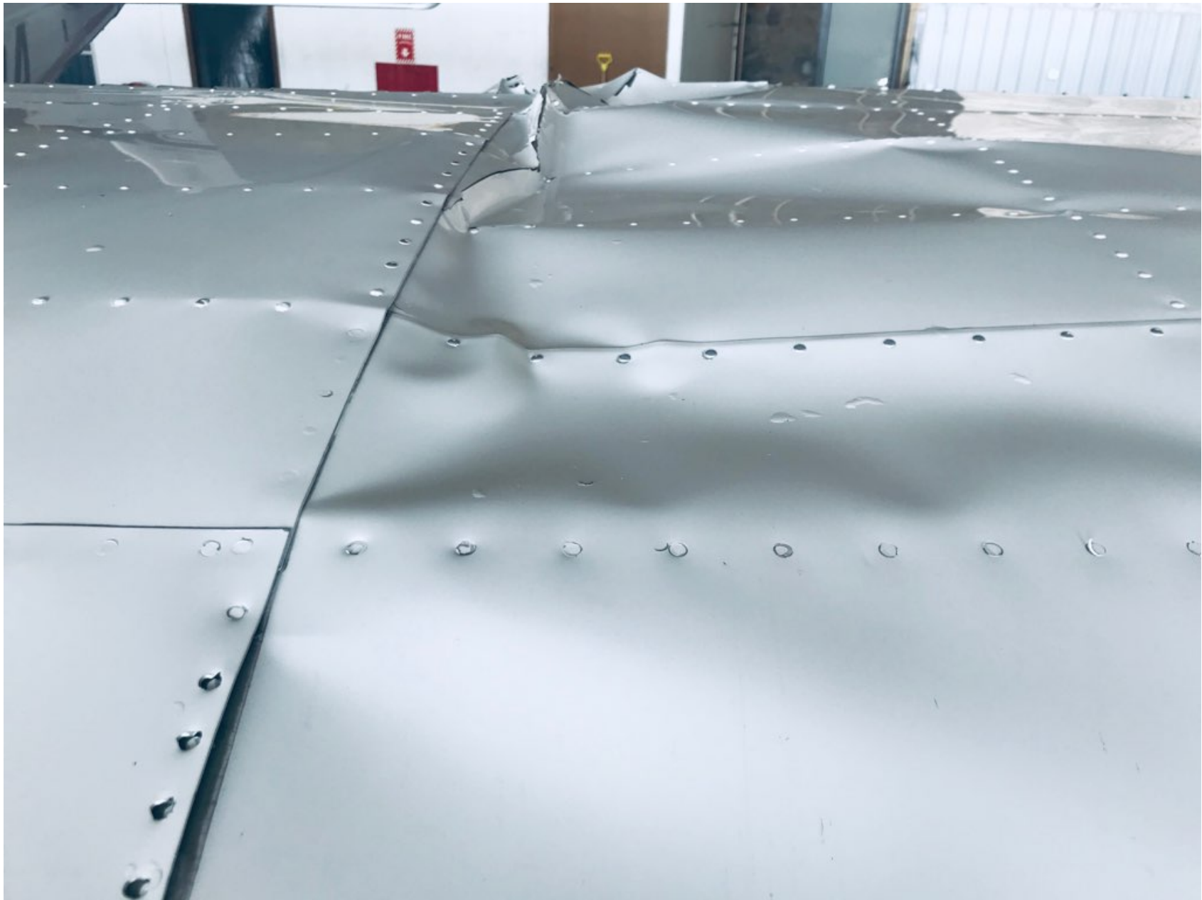
Photo 3 – Left Wing Damage (Airport Operations Photo)
