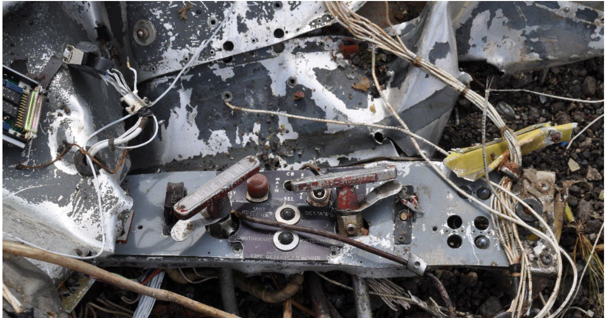
Figure 8 - Engine Fire Control Panel
