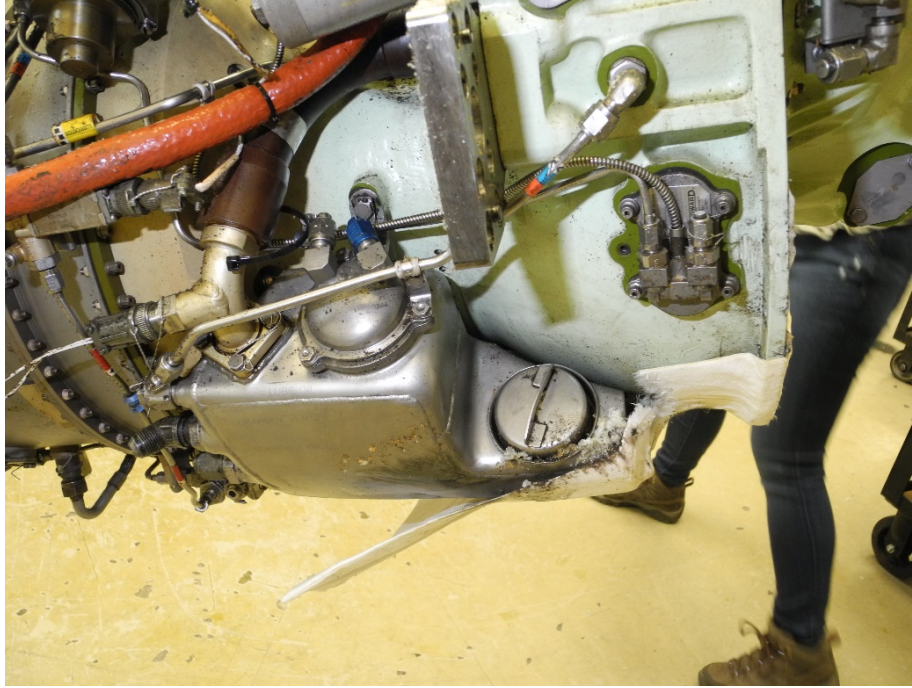
Photo 8 – Oil Tank – Still Installed on Engine
