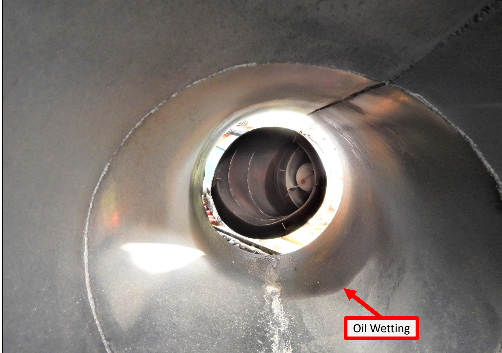
Photo 4 – Eductor Interior Surface (Photo Courtesy of Honeywell)
