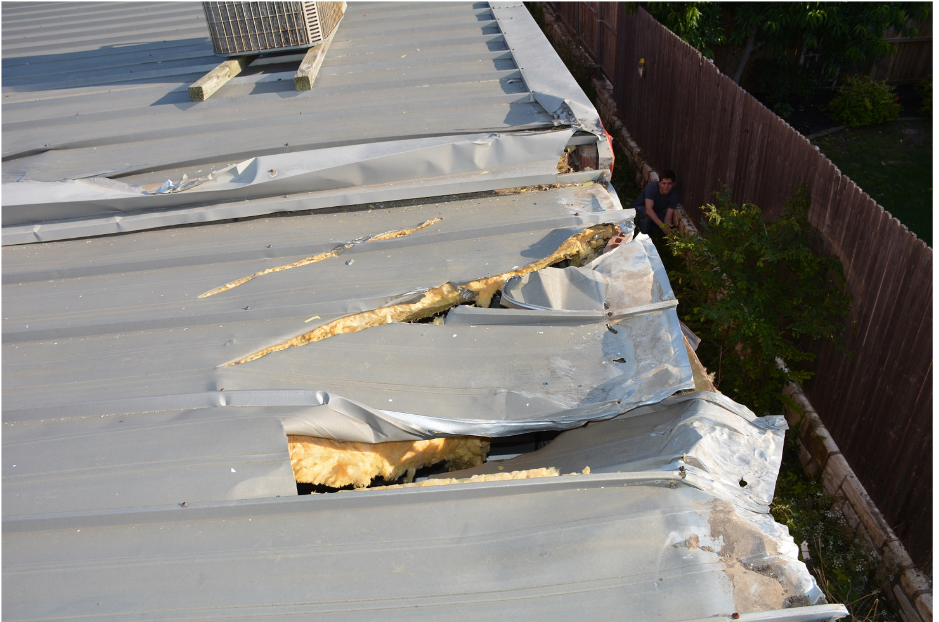
Photo 3 – Propeller Cuts
