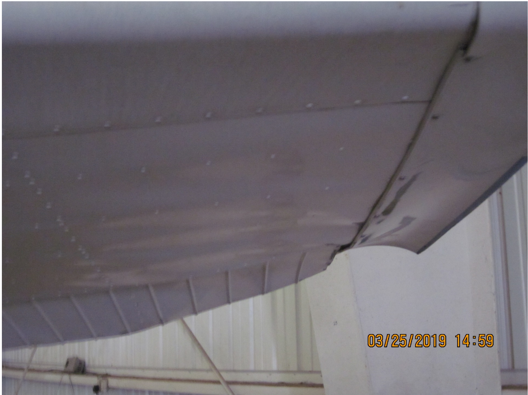
Photo 2 – Damage to Lower Skin of Left Wing and Aileron (Courtesy of FAA)
