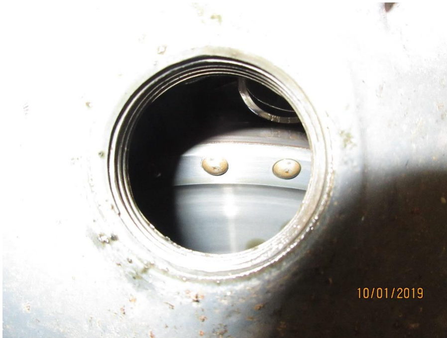
Nose Inspection Port – (*Note - Cam Hub Rivets intact) Photo #6
