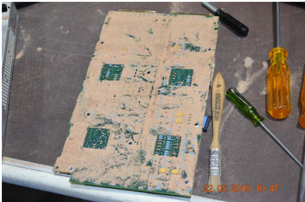
KC 225 – boards were removed for cleaning
