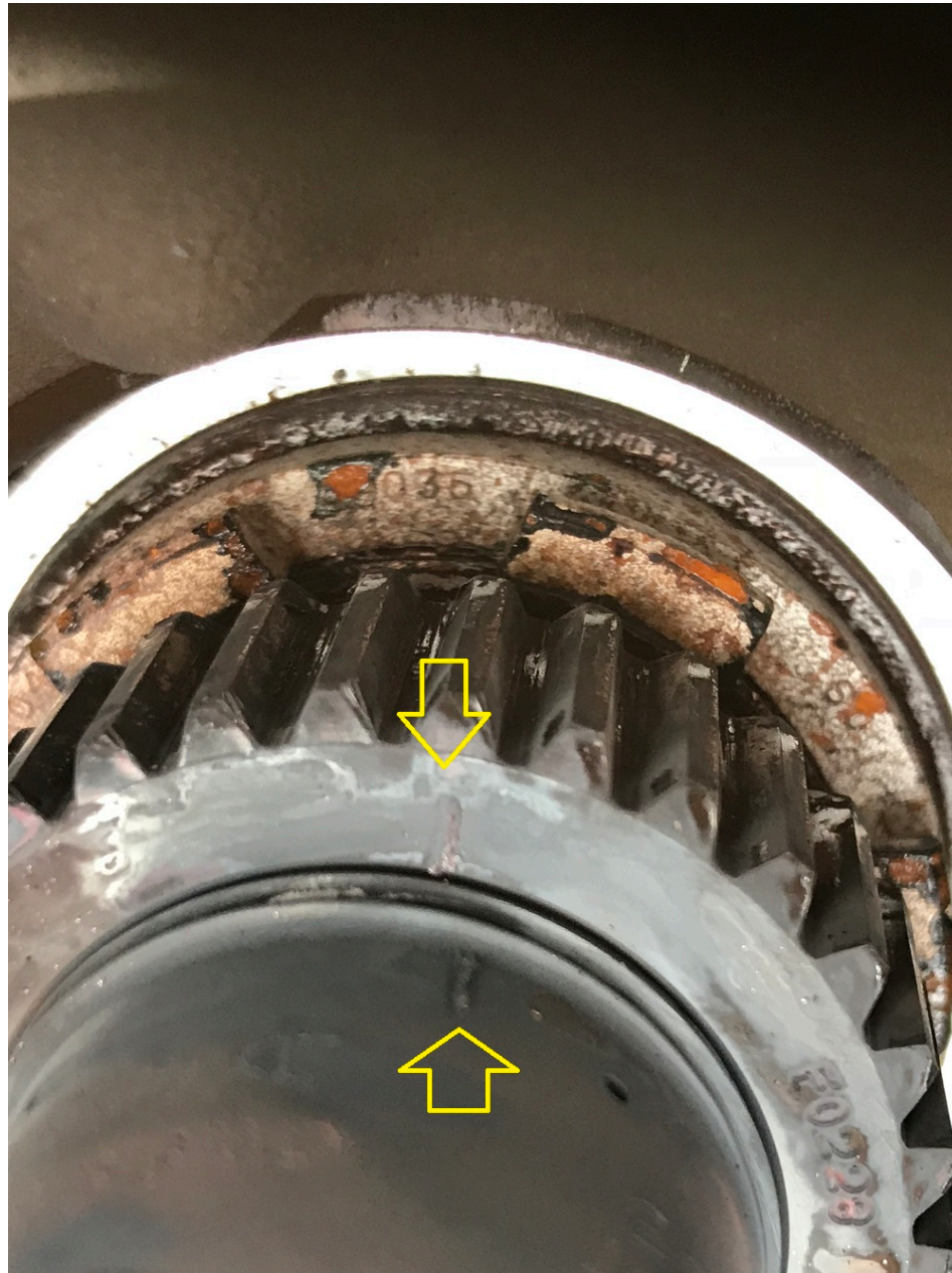
Photo 3 - Module 5, Slippage marks
