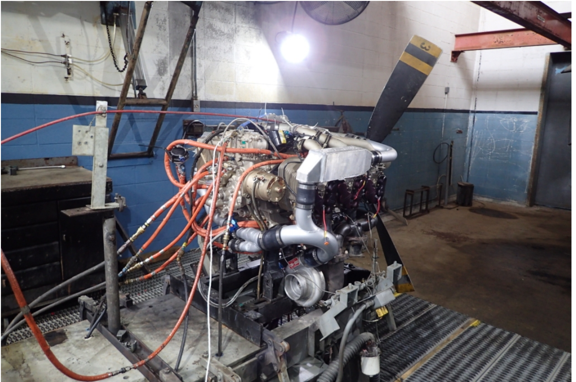
Photo 9 – View of the engine installed on the test stand (CM Photo)
