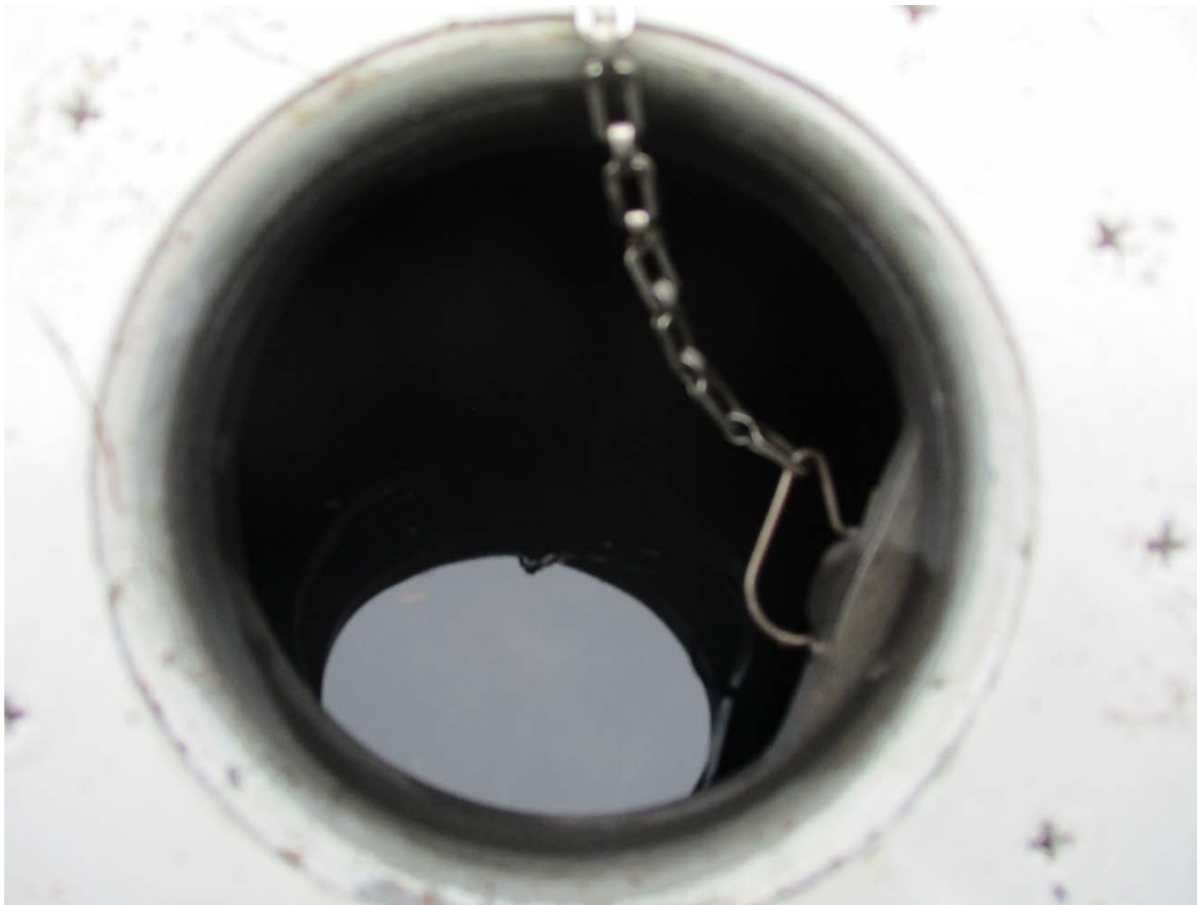
Photo 3 - Fuel (looking inside tank) photo courtesy of FAA
