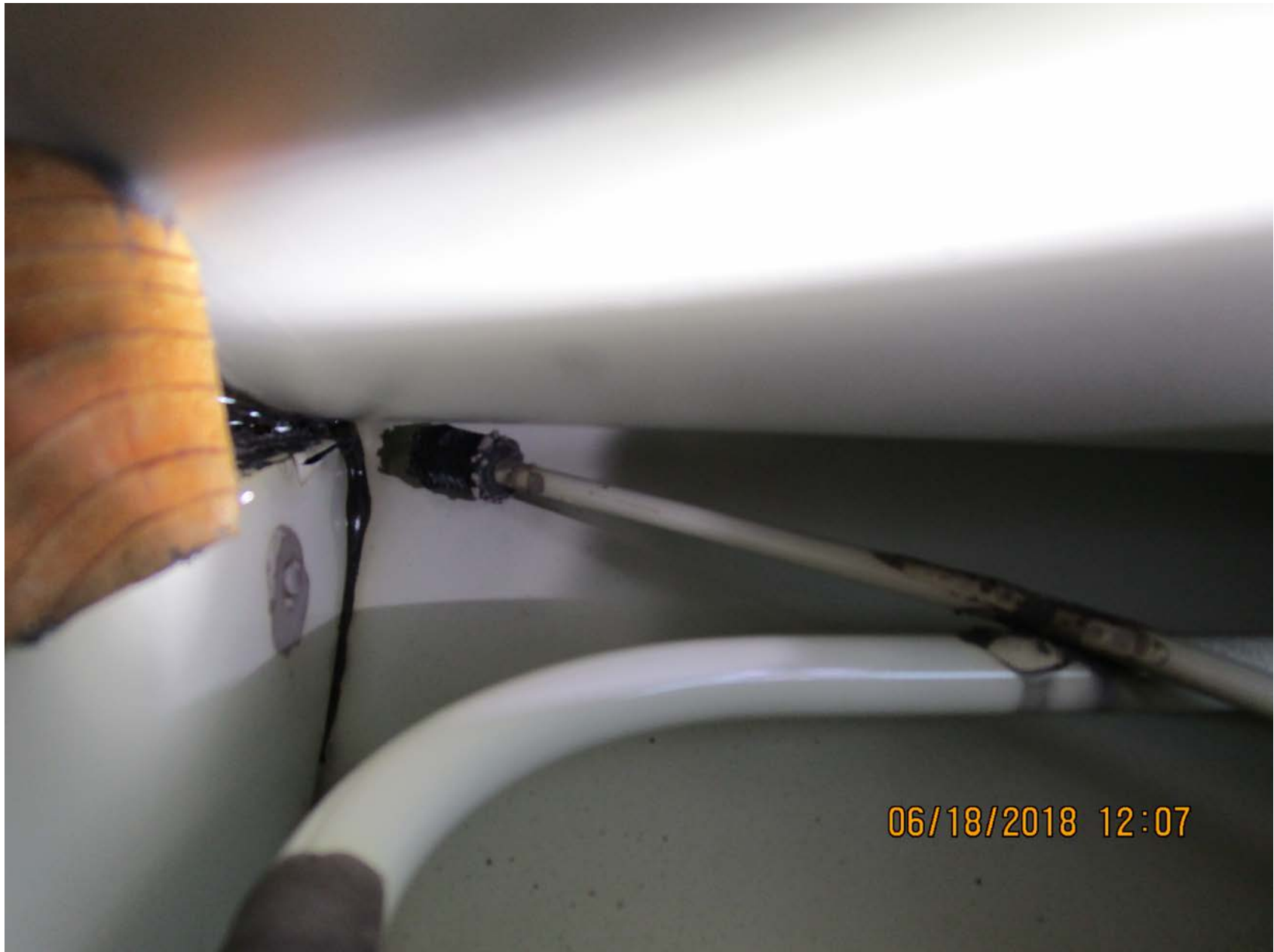
Photo 1 – View of small vent tube in outboard right wingtip (FAA Photo 1630)
