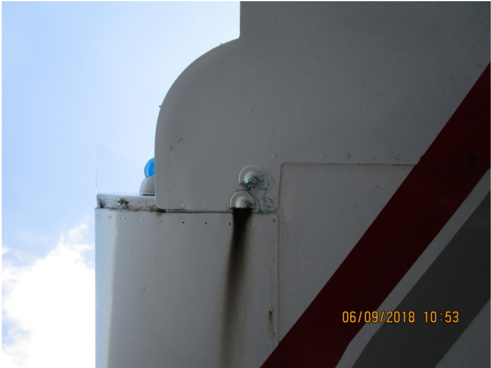
Photo 6 – View of soot and fuel stain under the wing near navigation light (FAA Photo)
