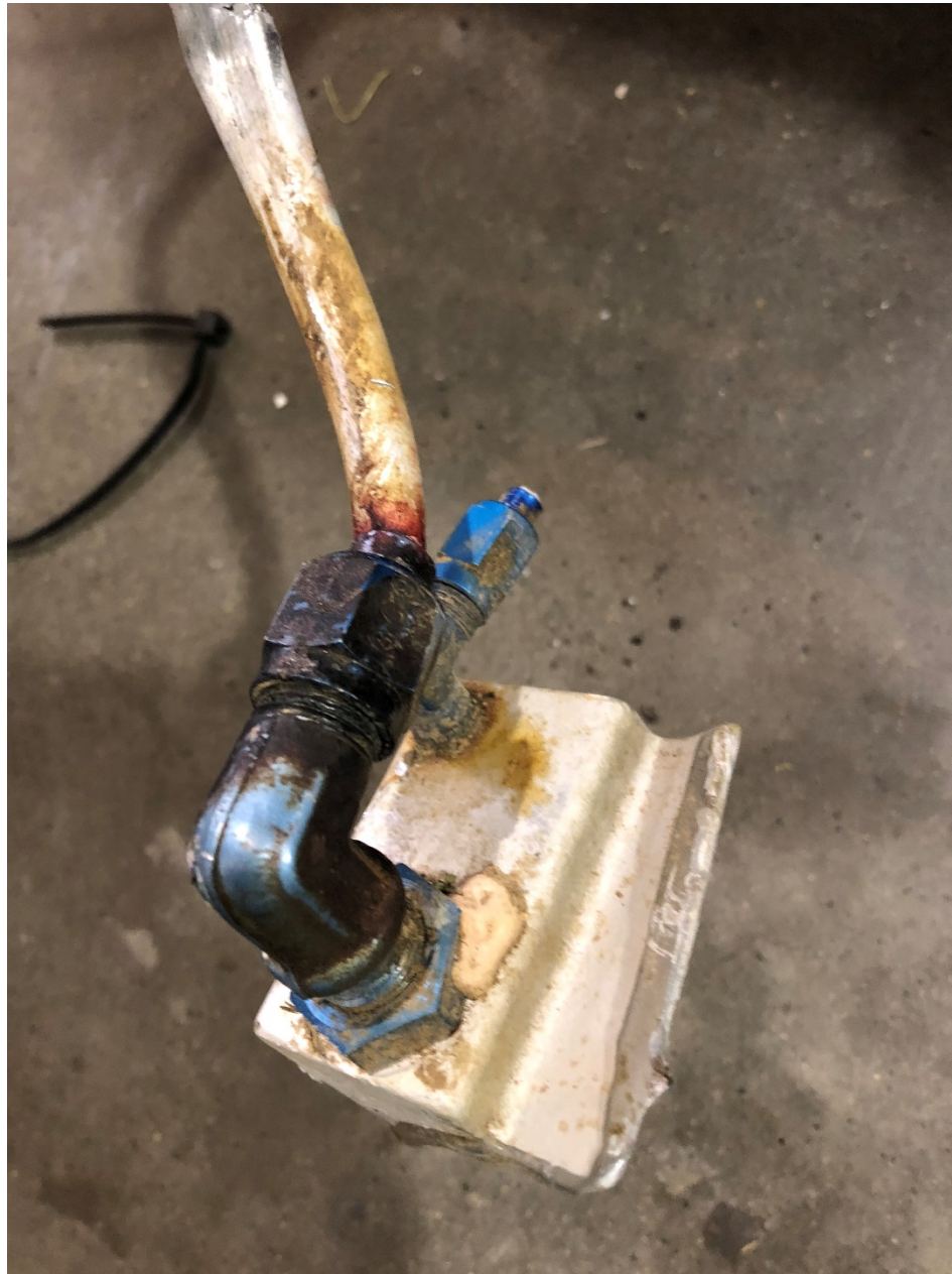
Photo 6 - View of fittings from the left fuel tank that exhibits staining.
