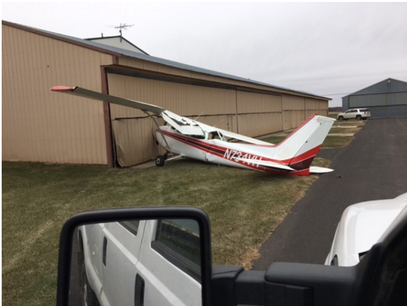
Photo 4 – Airplane Wreckage and Hangar
