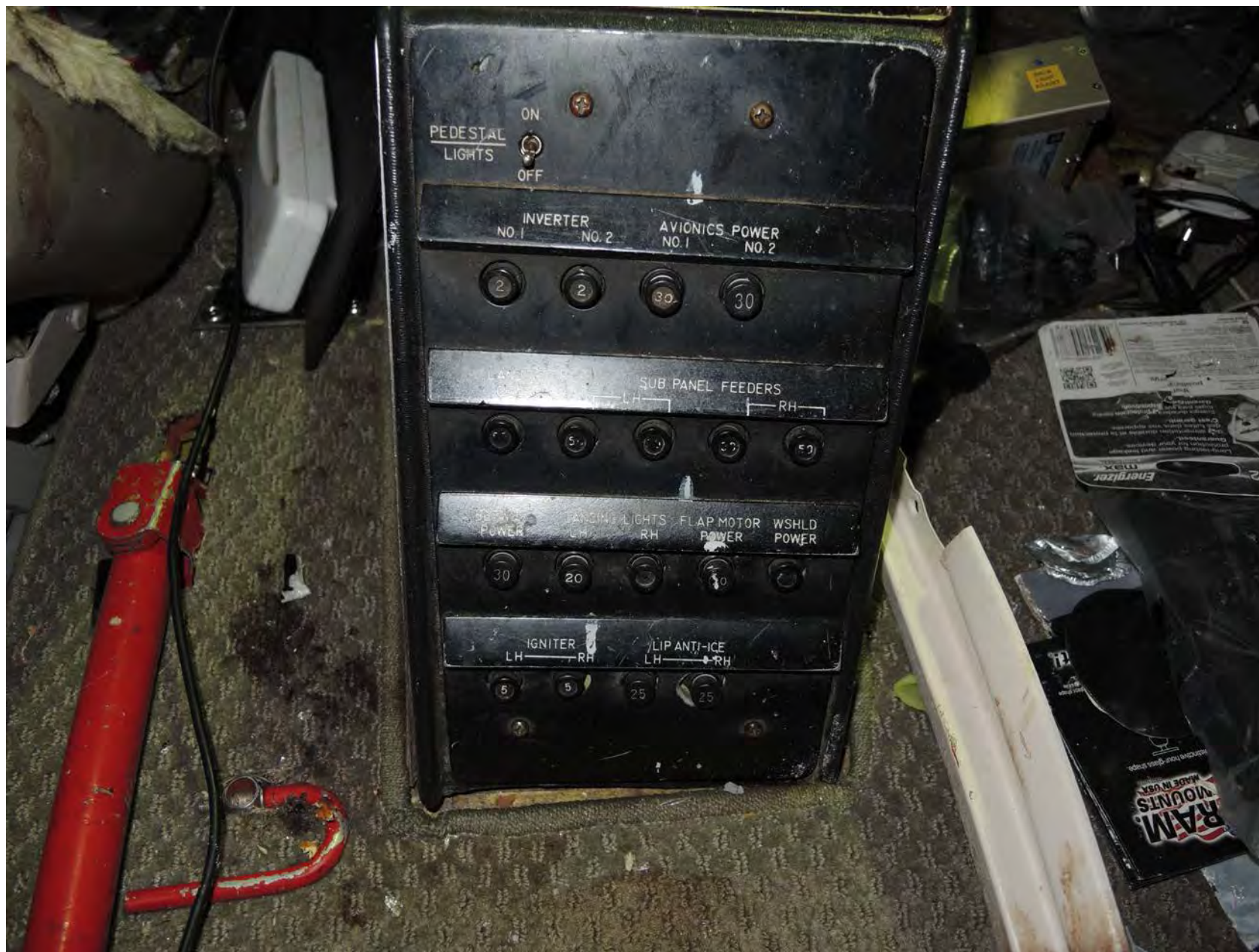
Photo 18 - View of the lower portion of the pedestal.
