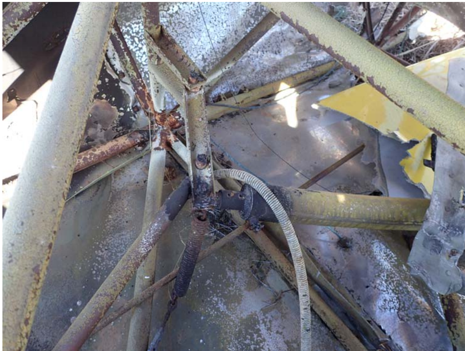
Elevator Controls at Rear Idler
