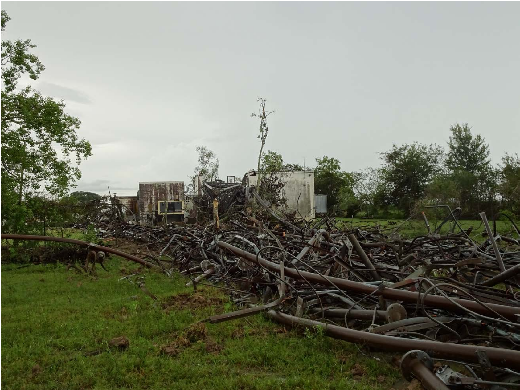
Photo 5 – Base of Tower after Collapse
