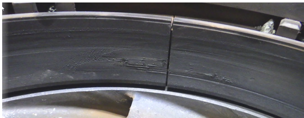
Photo No. 21: CT shroud rubbing
