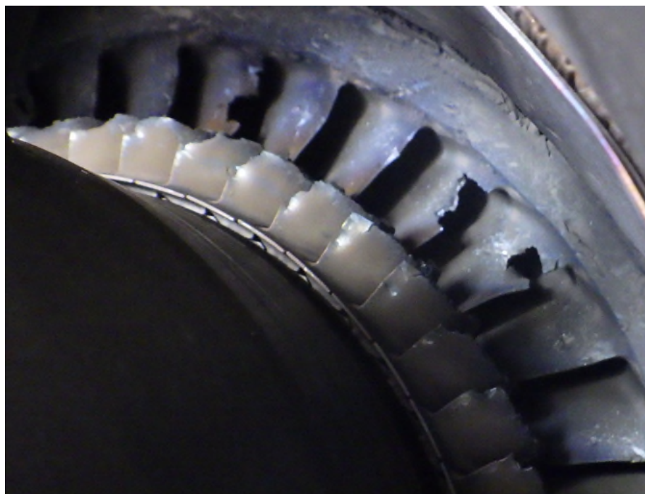
Photo No. 5: PT blades all fractured at \frac{1}{3} span
