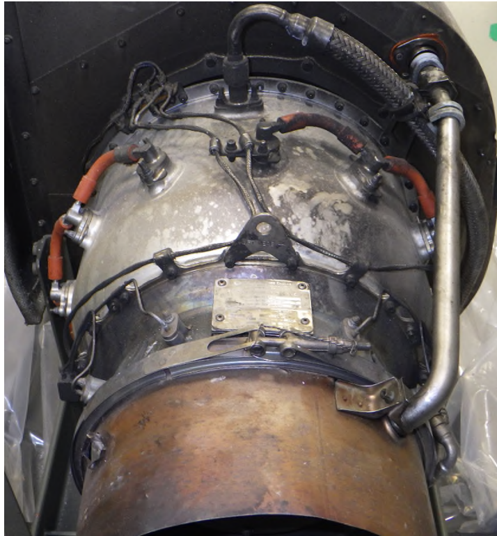
Photo No. 46: Soot residue on BB0045
